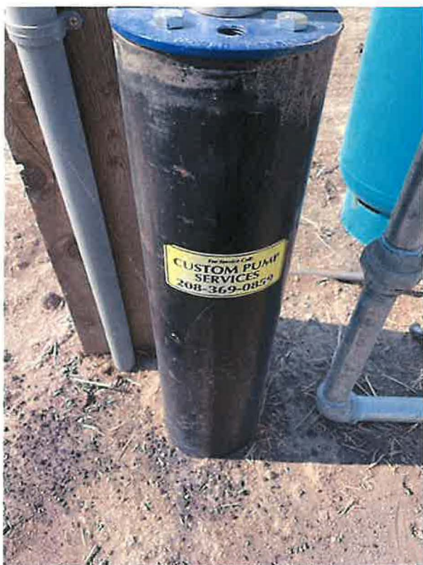
Figure 5. Photograph of the external well casing. Could not see the tag number because an additional casing was added on over the original casing.
