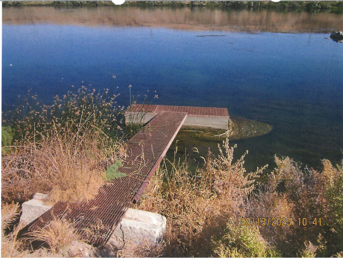
Figure 1. Causeway to intake from Snake River.
