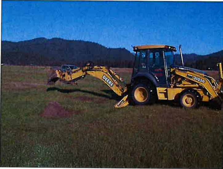
Figure 16. Backhoe used in soil pit excavation (Soil Pit 1).
