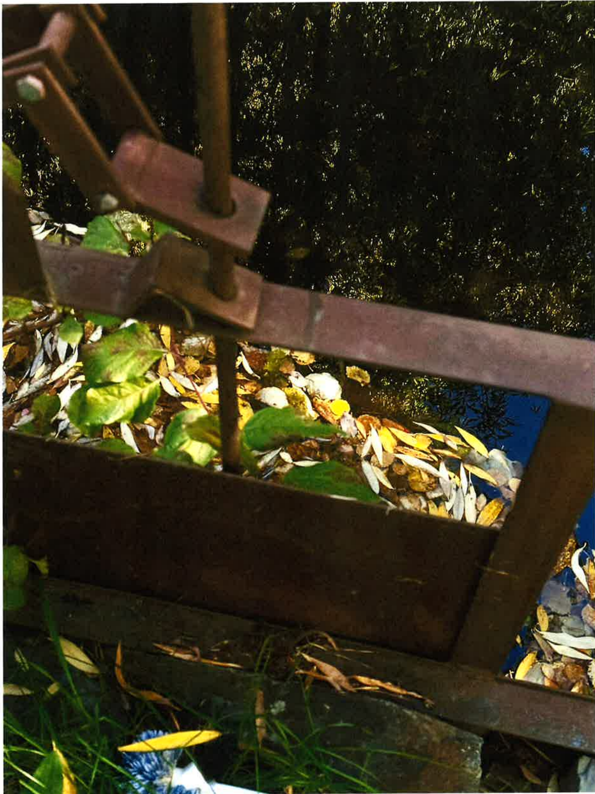
Diversion Headgate from Fourth of July Creek
