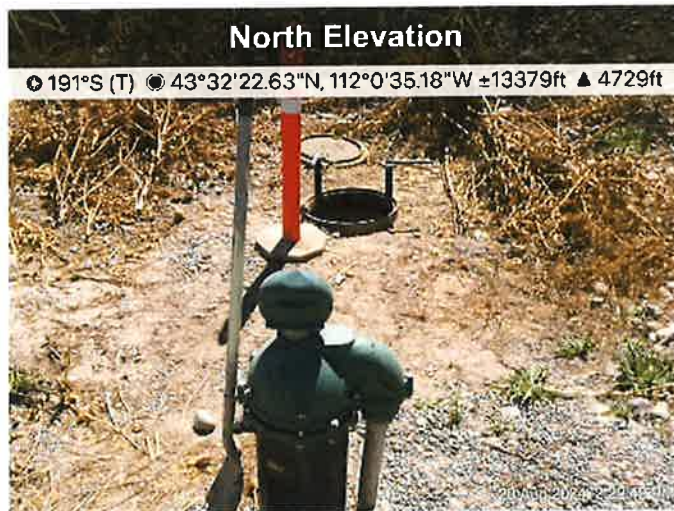
Well and manhole
