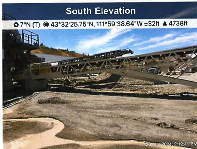
conveyor for gravel wash station
