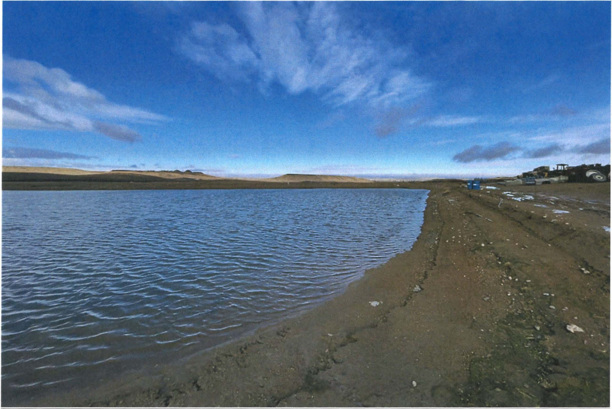
Figure 8 Storage pond located in 02N 04W SWNW \frac{1}{4} of Section 28. Pond stores both ground and surface water.
