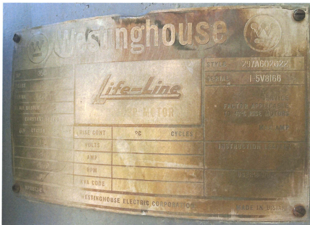
Figure 6 350 hp pump from Westinghouse with motor serial number I-5V8166.
