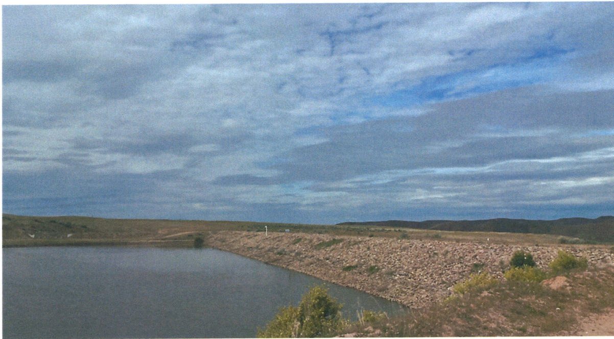
Figure 3 Earthen Dam on the western end of reservoir. Hydraulic headgate is located within the dam.
