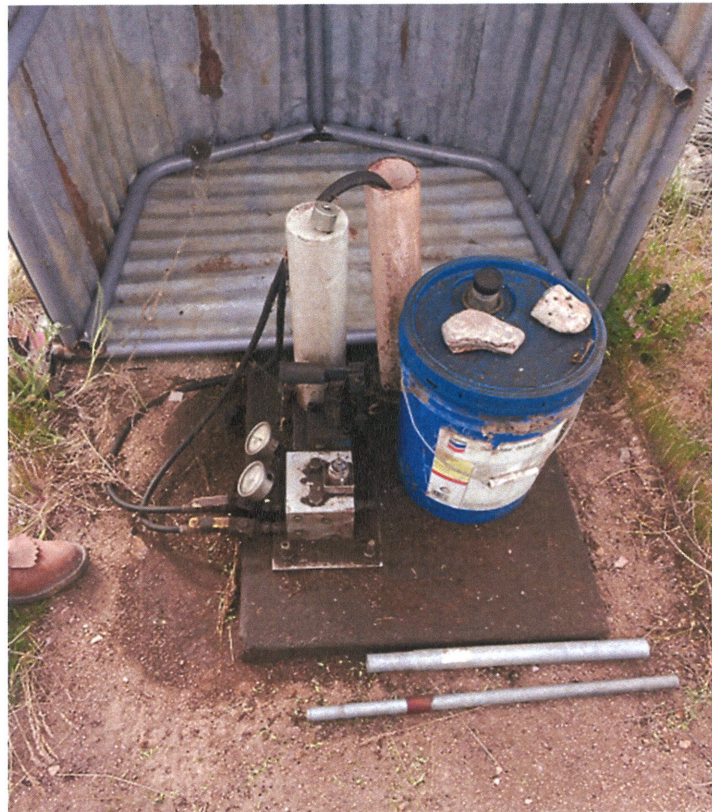
Figure 9 Hydraulic headgate diversion located on the earthen dam at the west end of the reservoir.
