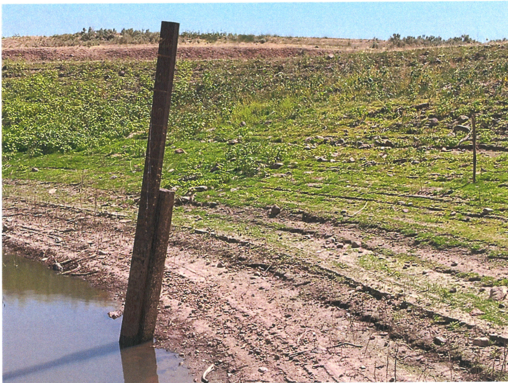
Figure 5 Staff gage used to measure reservoir capacity, at current reservoir level at the time of a dam inspection.
