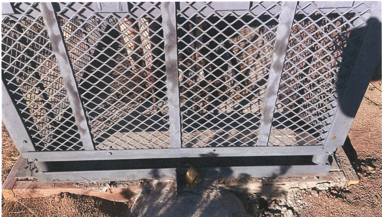
Figure 10 Lockable device installed to the headgate cover after the field exam.
