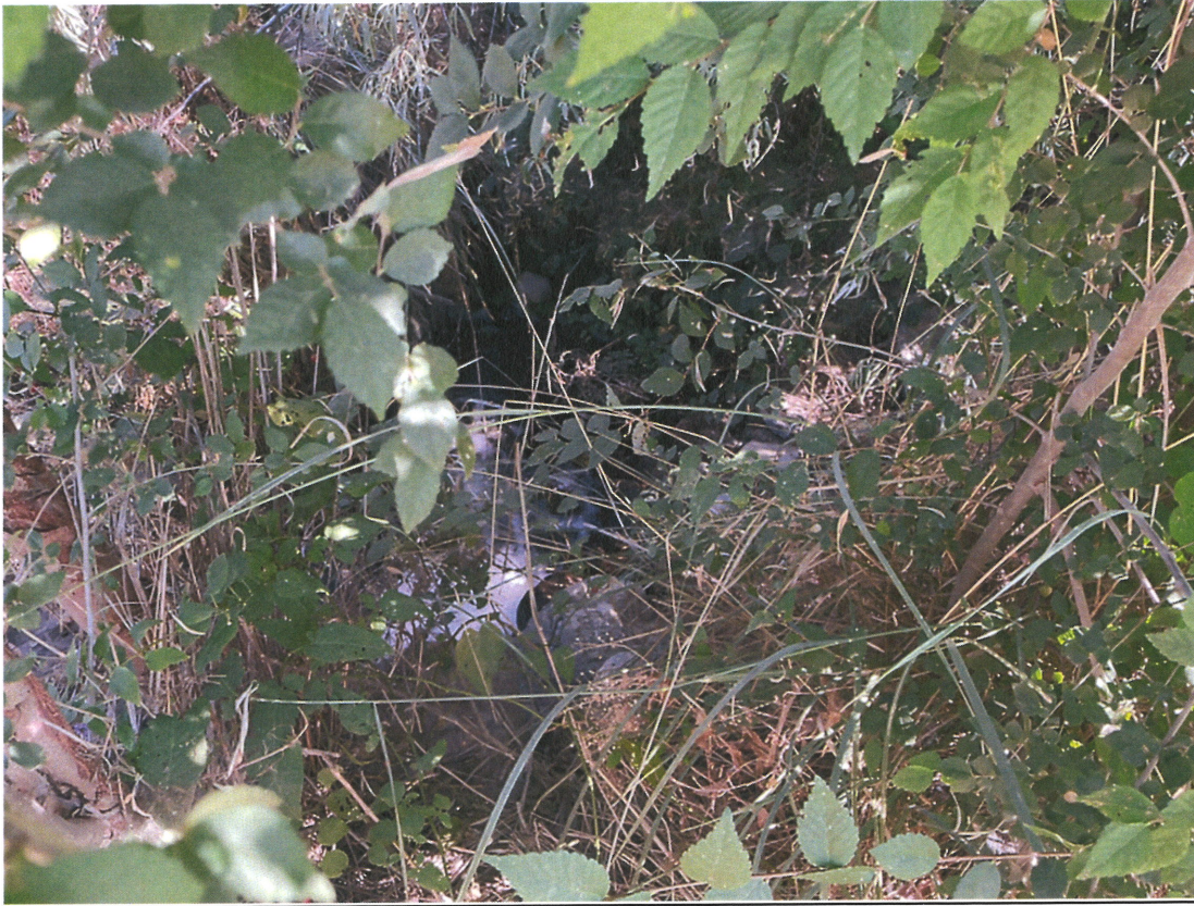
Figure 3 Outlet of the 12" culvert, returning water to the ditch that then returns irrigation water to the Snake River.
