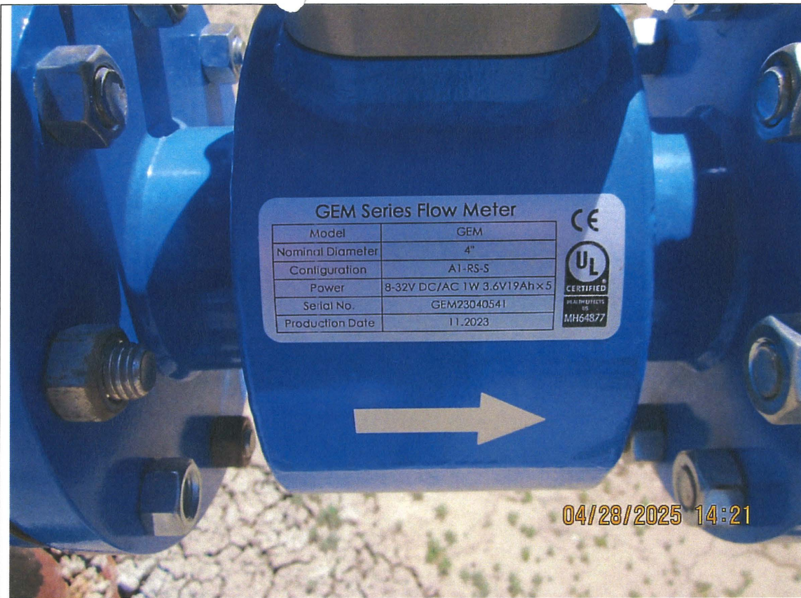
Figure 3. Closeup of GloTech flowmeter model GEM.
