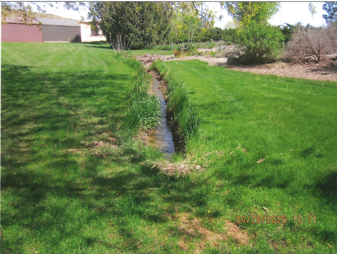
Figure 14. A section of one of the ditches connecting the ponds.
