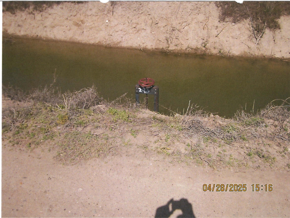
Figure 7. Headgate at A-Line canal, showing where surface water is diverted to the ponds.
