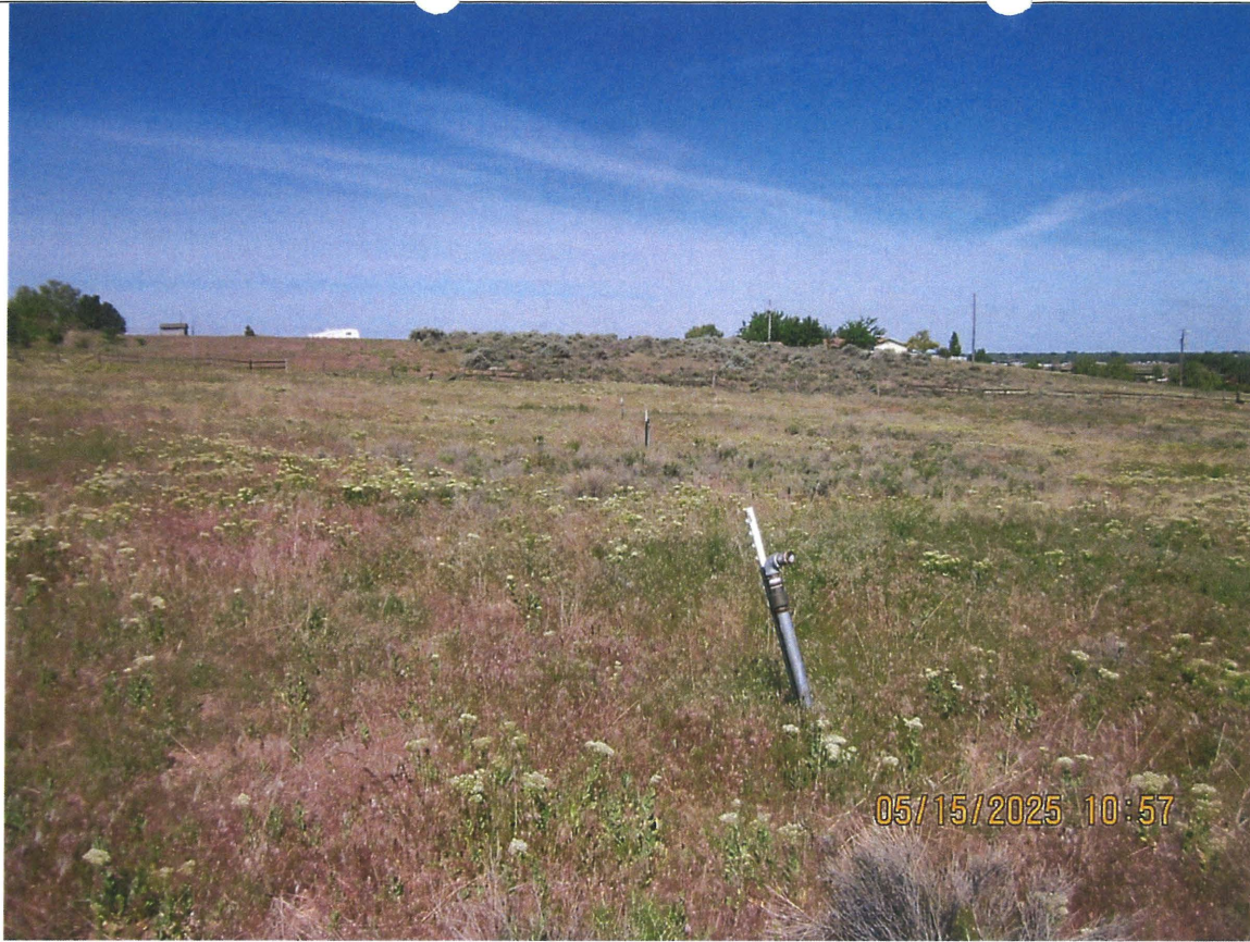
Figure 7. Three dust abatement valves.
