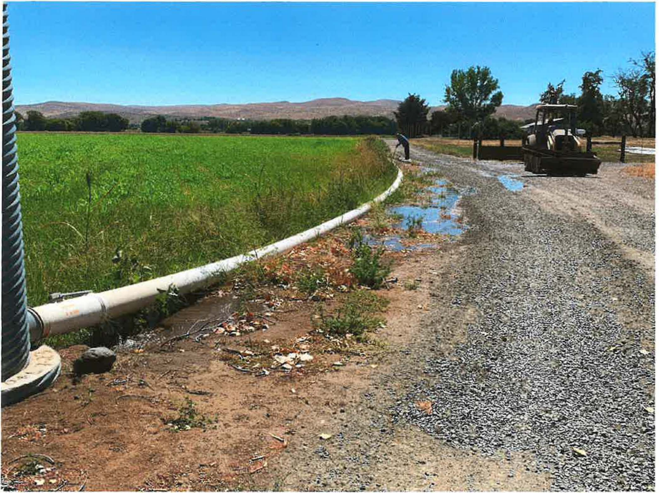
Beneficial use. Irrigating via gated pipe.
