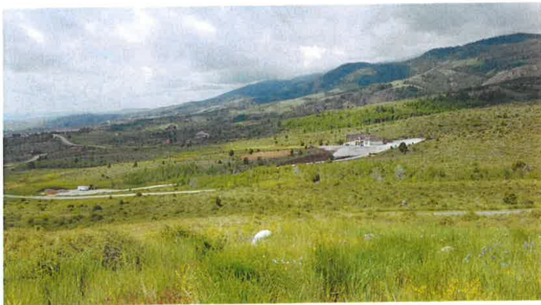
Development that has occurred at Sam's Hollow Water Company as of 2018
