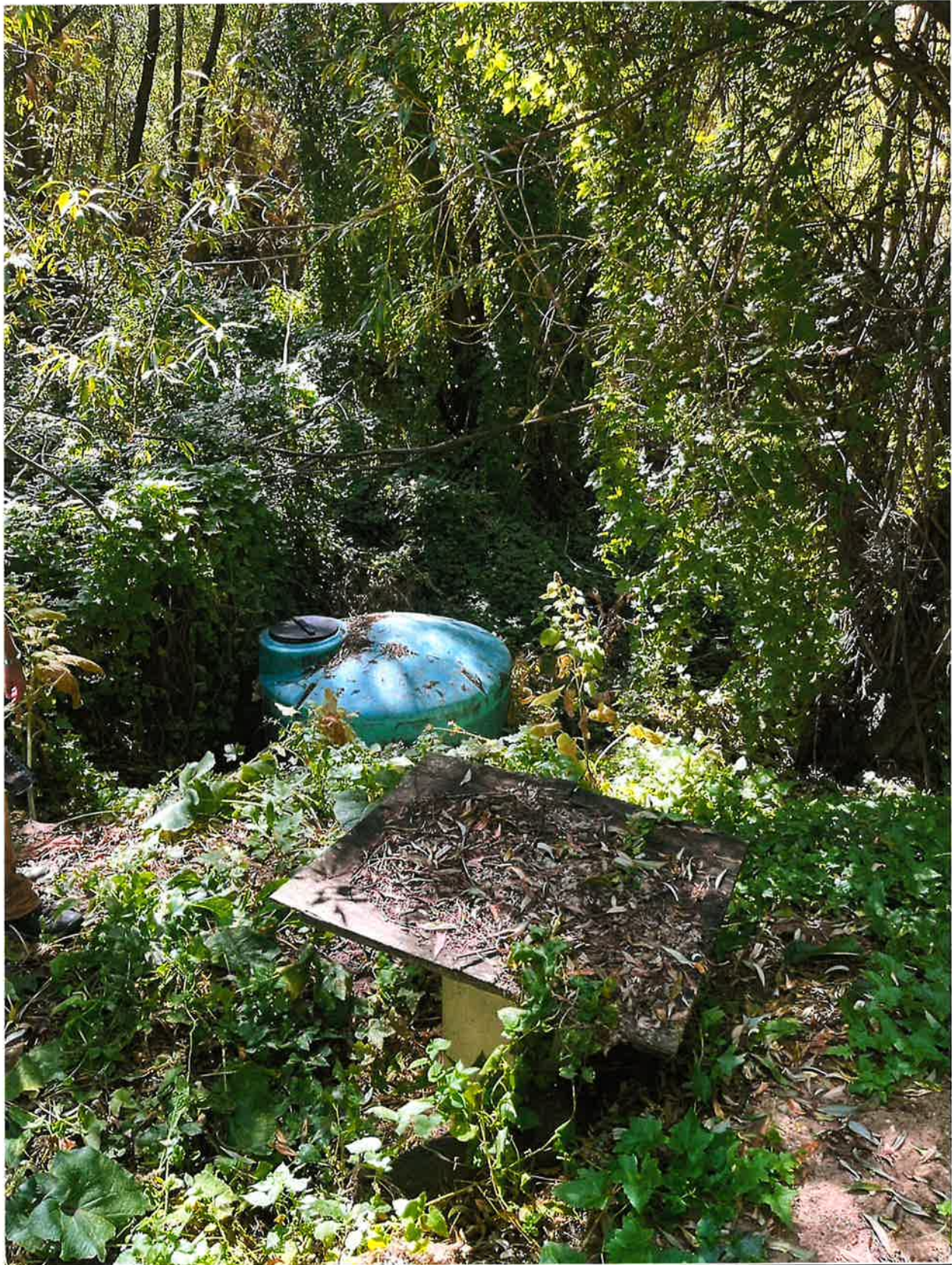
Figure 2 Diversion infrastructure looking south.
