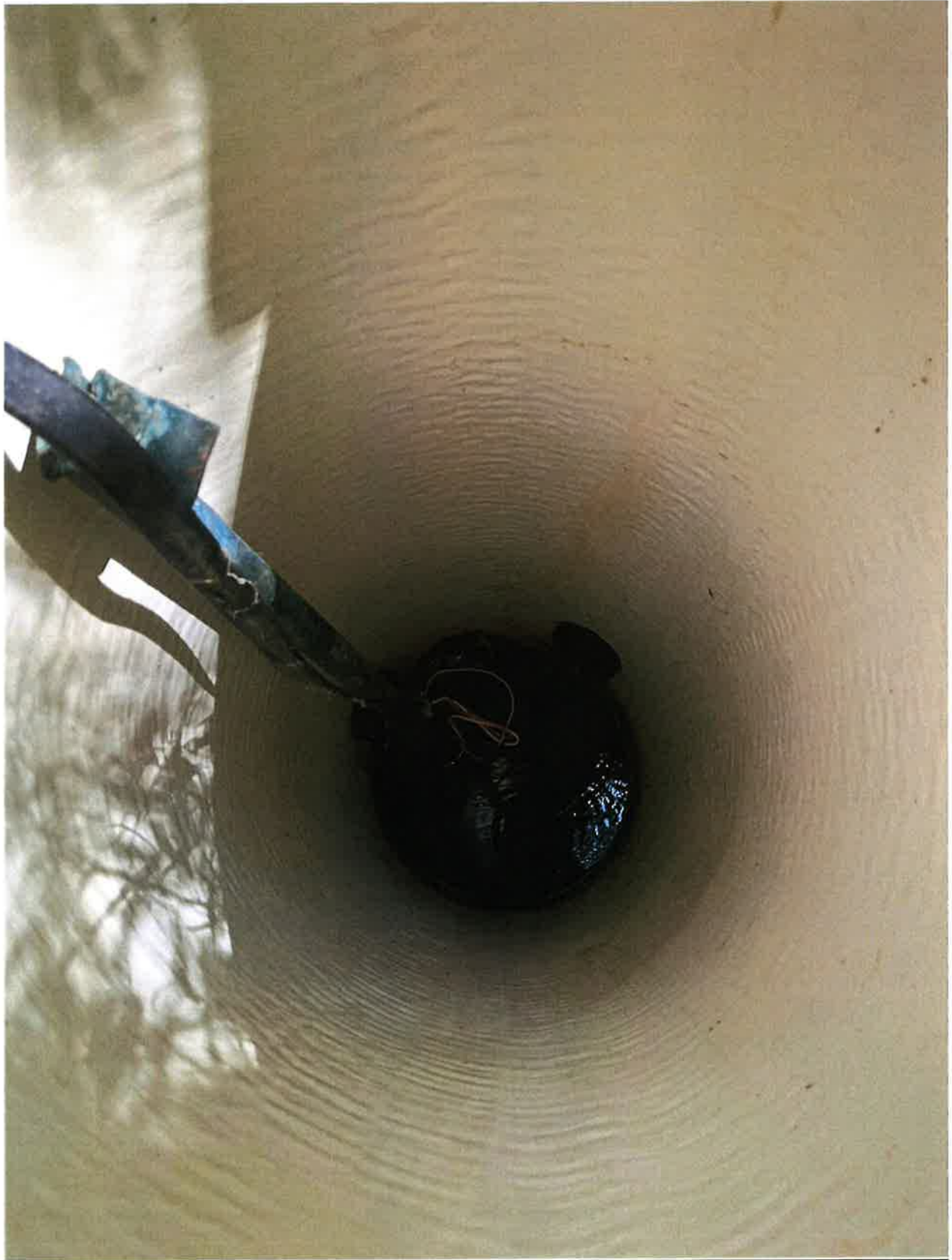
Figure 5 View of water in pipe.
