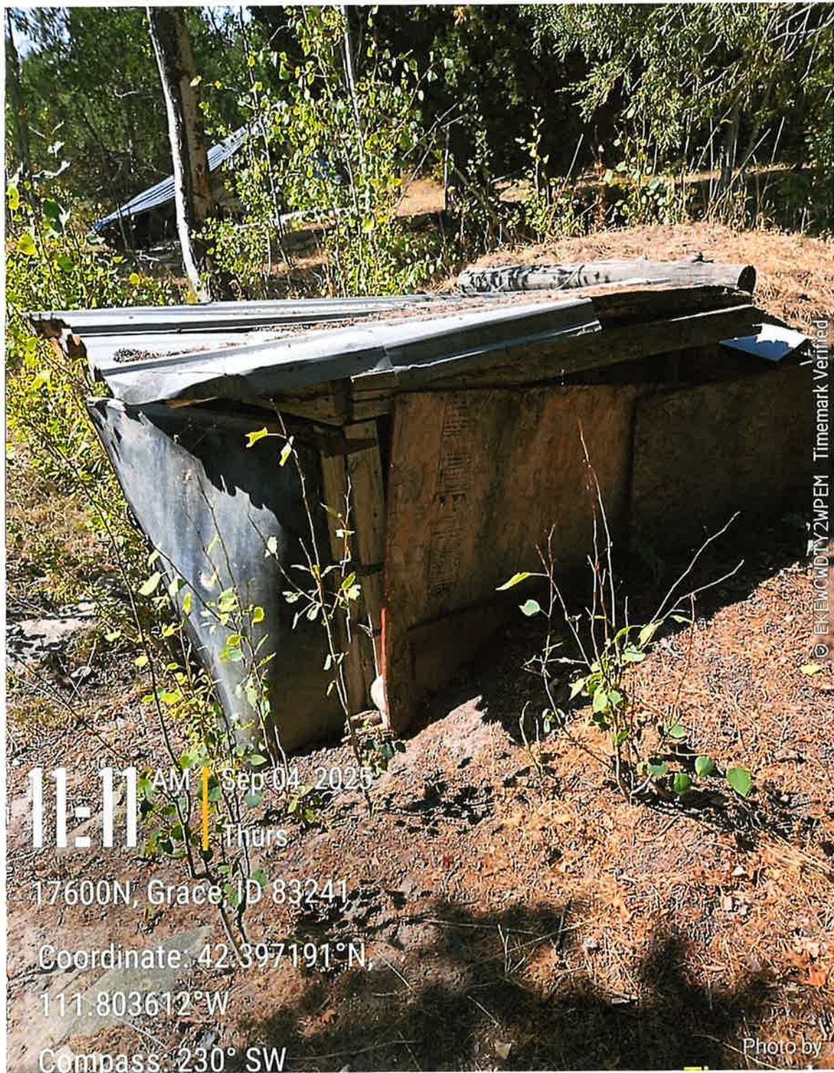
Figure 3 Structure "protecting" the spring
