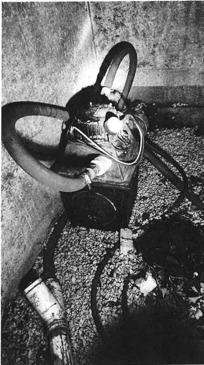
Turbine with catch basin to collect water to spillway back into fall creek
