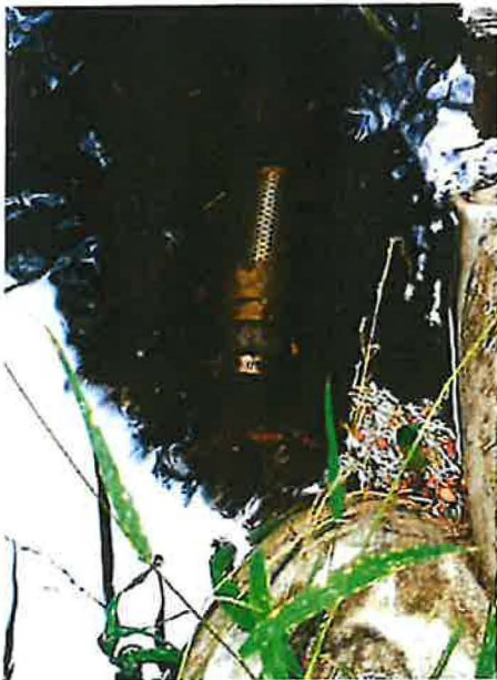
Intake in creek bed - Photo of completed work attached to Statement of Completion for Submitting Proof of Beneficial Use
