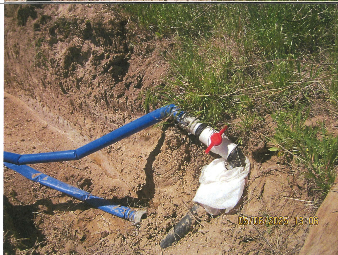
Figure 4. Close up of 4-inch pvc valve.
