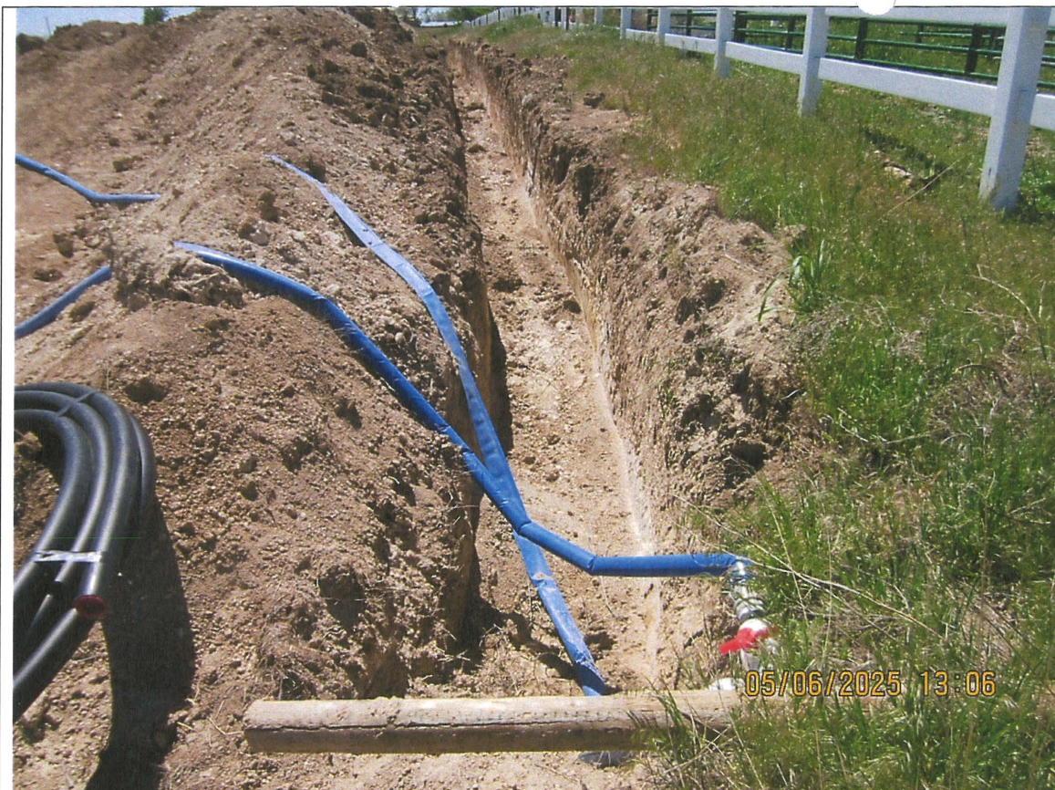
Figure 3. Blue lay flat hose coming off of pvc valve and going to sprinkler. Also, new trench extending up fence line.
