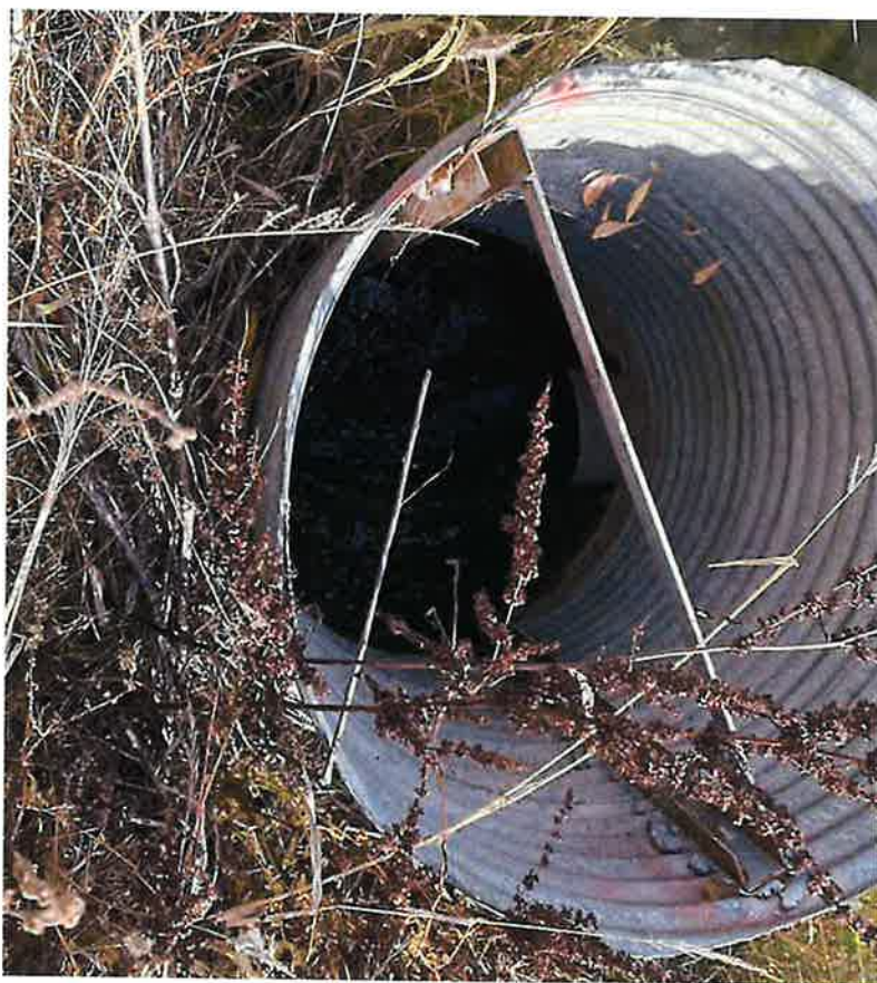
Outlet structure at Beaver Pond
