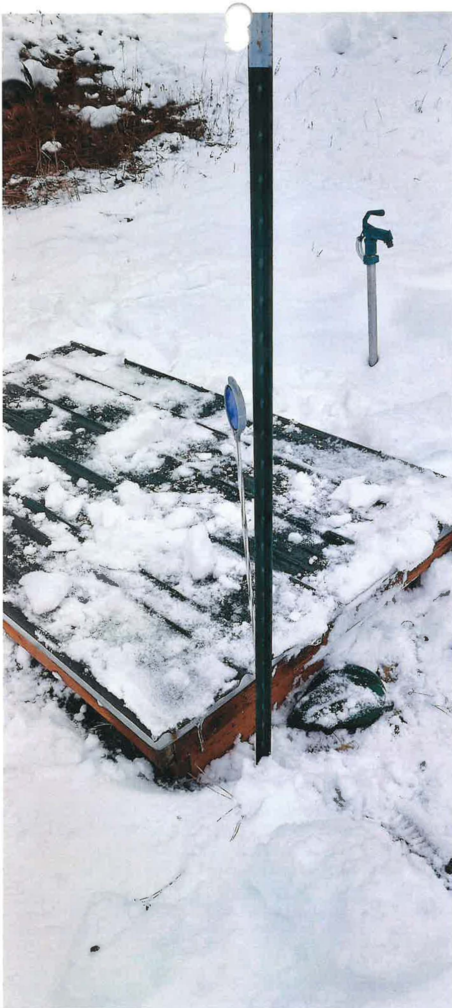
McCalmant Well Vault Cover Permit 91-8039
