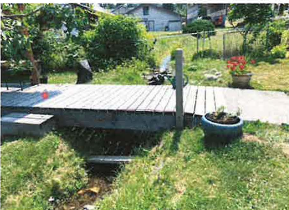
Bridge over the creek is 2.5 ' above high water.
