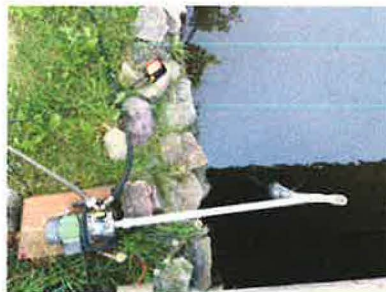
THE PUMP is located on the north-west side of the pond bridge. A mesh screen surrounds the intake pipe where it is located under water.
