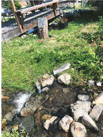
3" pipe with 1/4" screen cap at diversion intake point. Pipe is partially covered with rock at creek location and buried underground between creek and pond.
