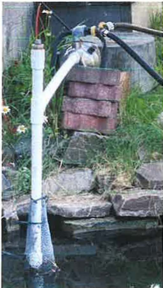
THE PUMP is located on the north-west side of the pond bridge. A mesh screen surrounds the intake pipe where it is located under water.
