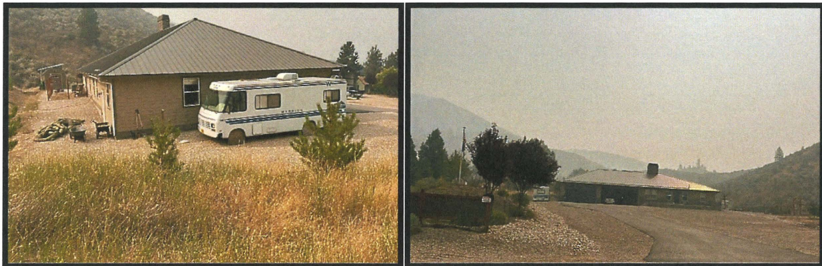
Photos 21 & 22- Lot #9, at 9 Red Fern Place.
