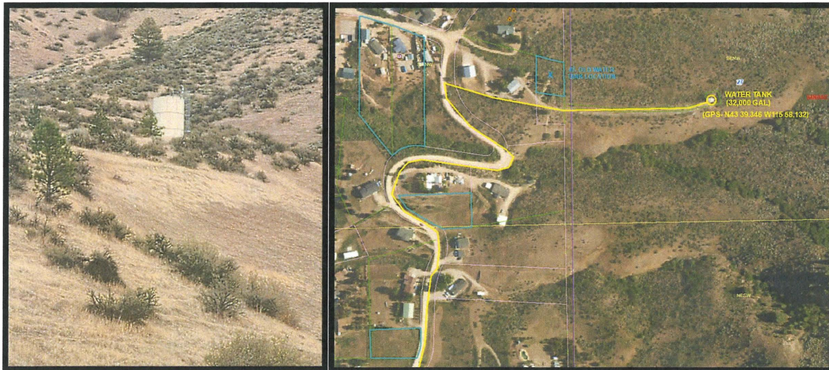
Photo 13 (Left)- The 32,000-gallon water tank northeast of the permitted place of use. Figure 2 (Right)- The parcel in the northeast of the POU is the original location of the water storage tank which was later moved to its current location uphill to the east of the POU.
