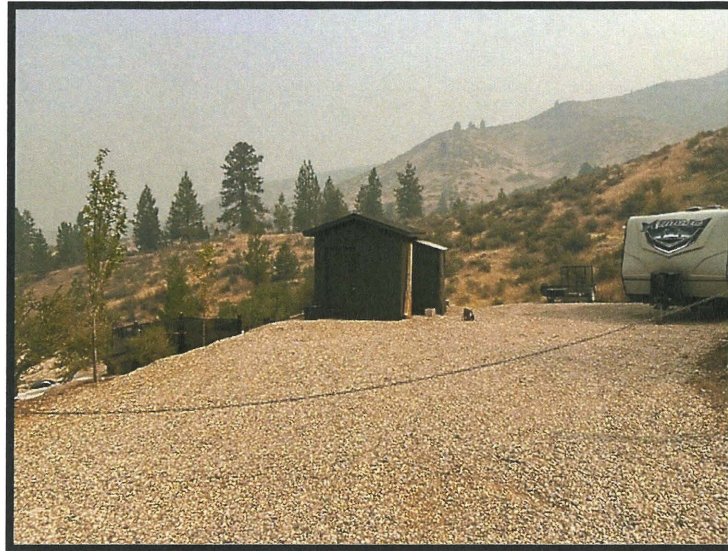
Photo 12(above)- Well #4 in the SWNW of section 27. The well has been abandoned due to contaminant levels. The well head has been crushed.
