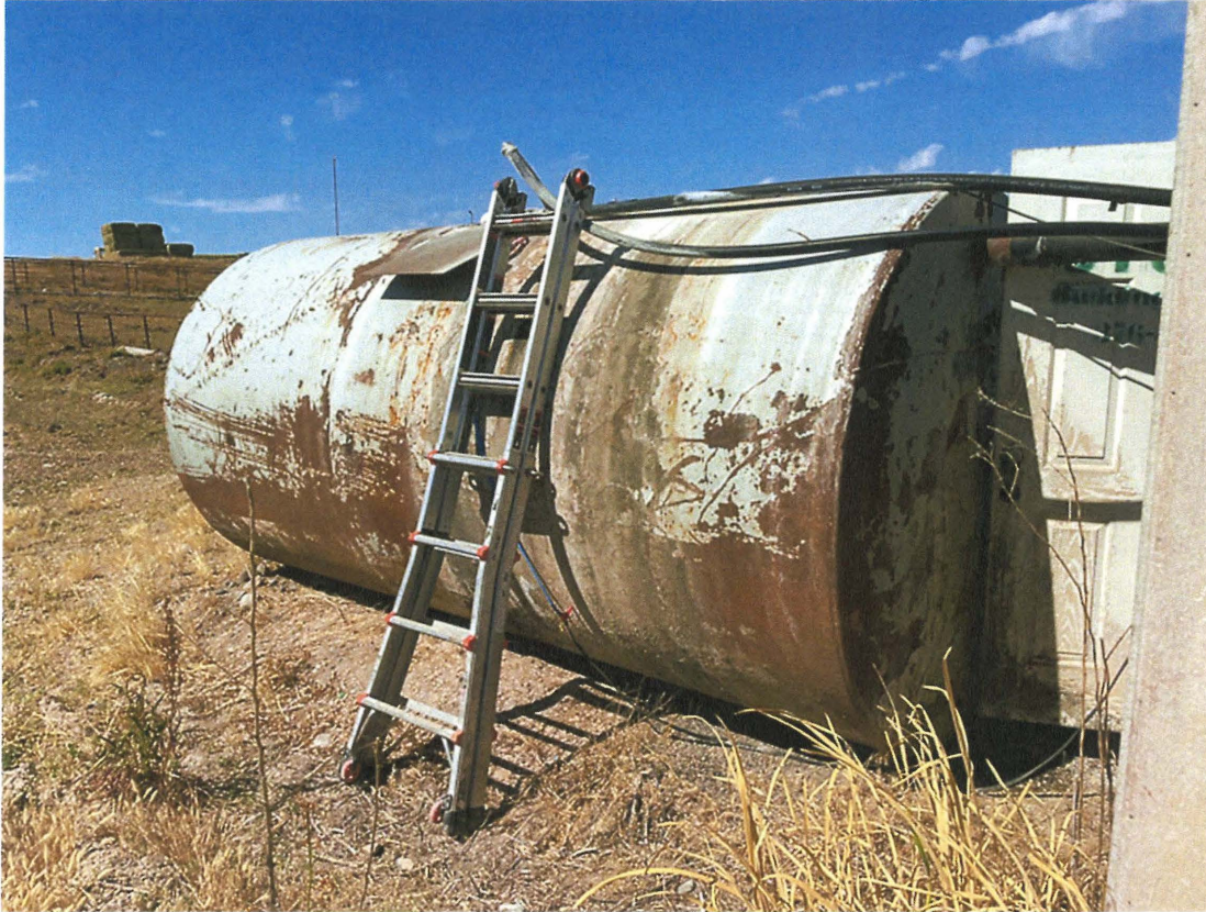
Figure 4 Storage tank with a 3,000 gallon capacity. The 1.25" water line is featured, running along the top of the tank where water is diverted to the tank.
