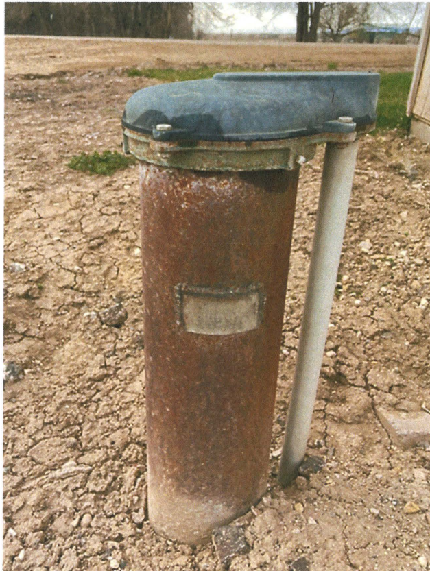
Figure 7 Well head for well 2, or D0031467.
