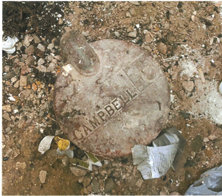
Figure 15 Well 5 well head, no metal tag number found.
