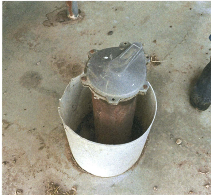
Figure 9 Well 3 with no identification tag.
