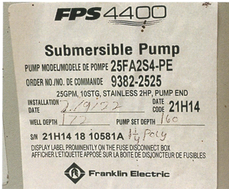
Figure 17 Well 5 pump specification tag showing 2 hp pump set depth, pump model, pump serial number, and installation date.
