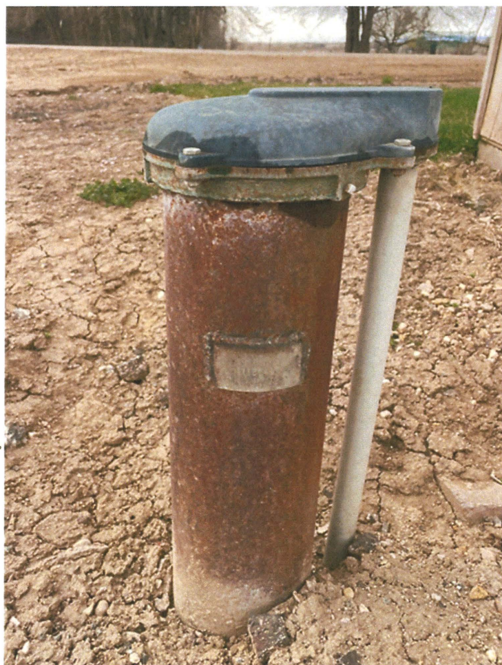
Figure 9 Well head for Well 2, or D0031467.
