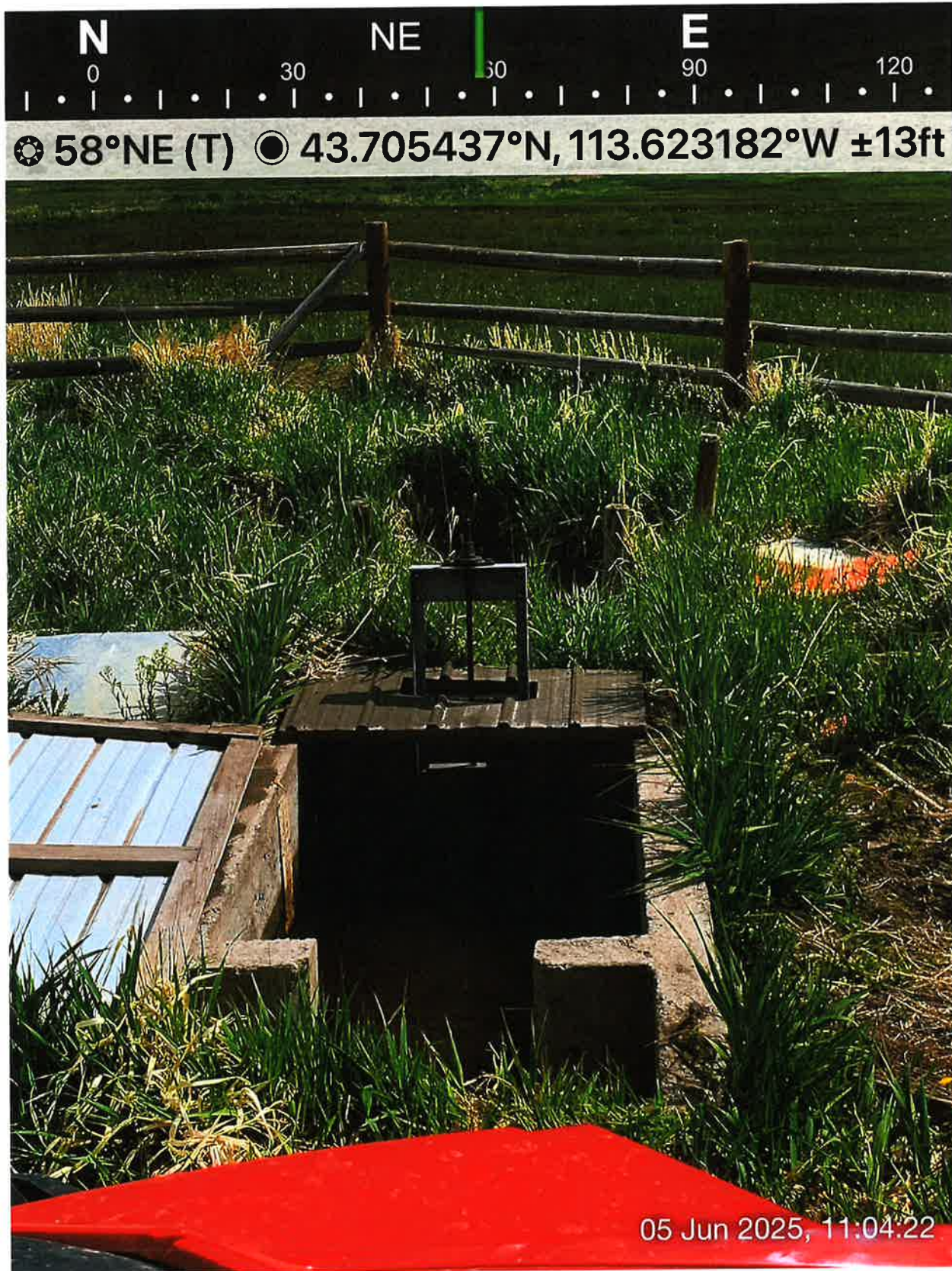
Headgate at inflow
