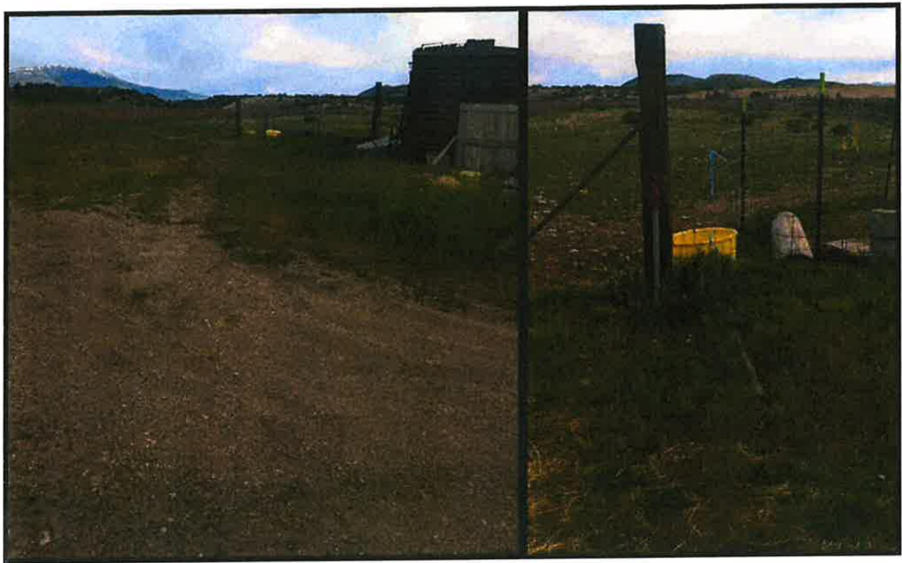
Figure 3. Stock water Pipeline Tee and Trough Hydrant, May 16, 2025.
