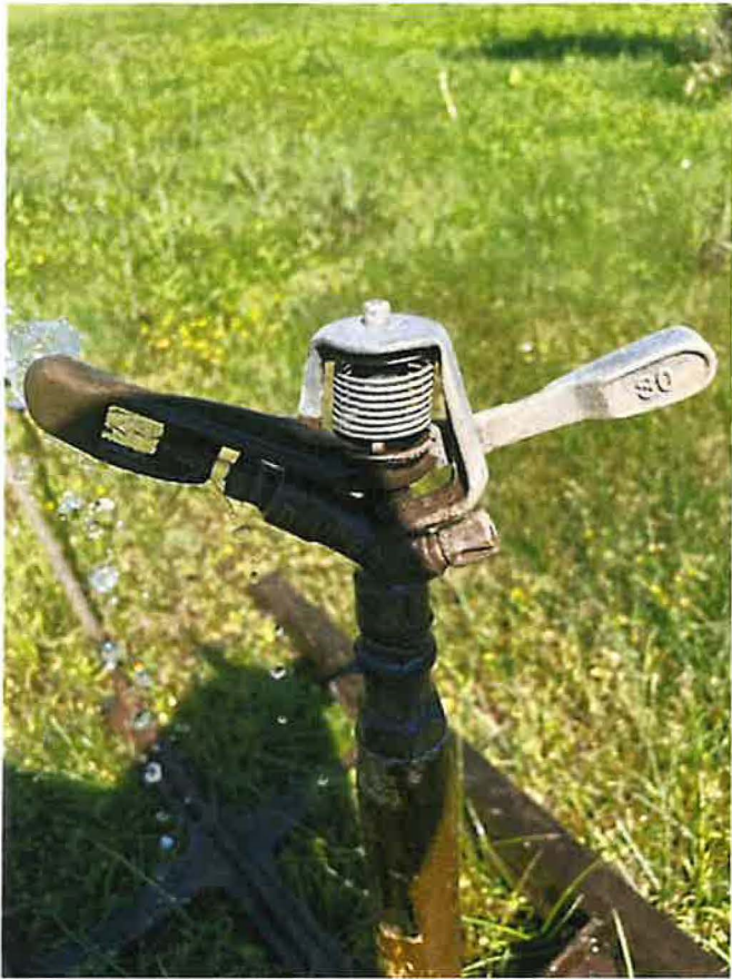
Figure 2: Sprinkler system with associated flow rates. Two sprinklers max are used at once
