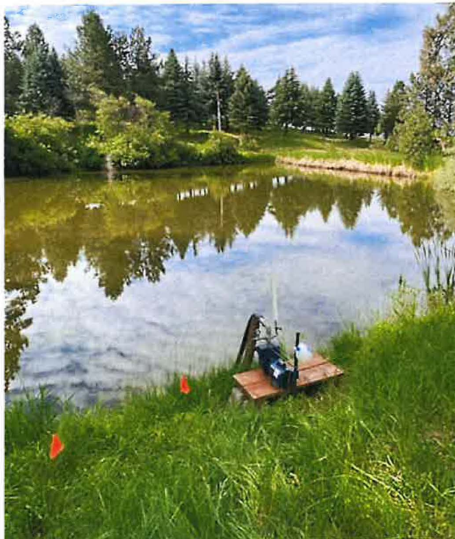
Figure 7: Lower pond with installed pump, facing south
