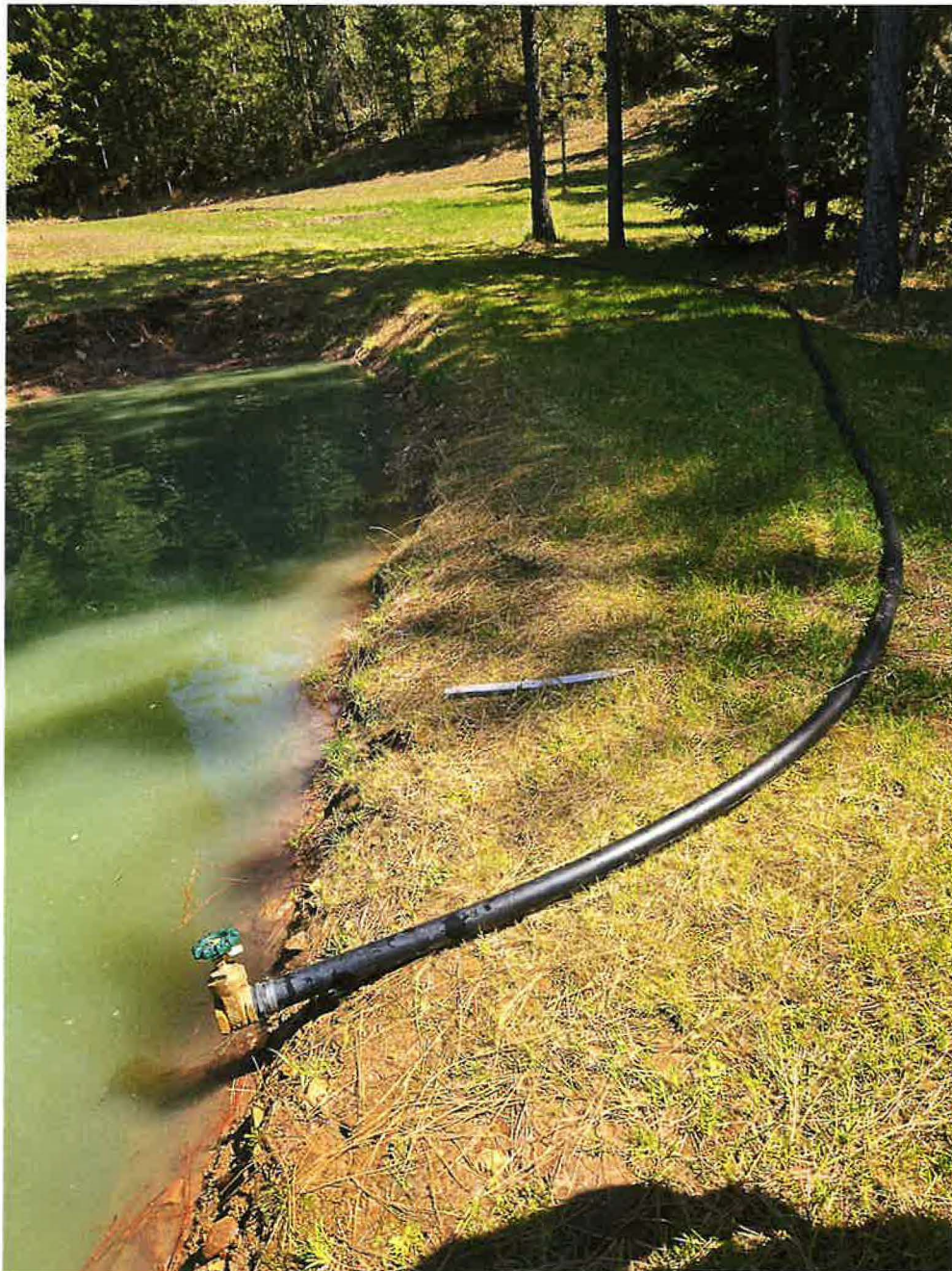
2 Inch Gravity Fed Line Diversion to Storage
