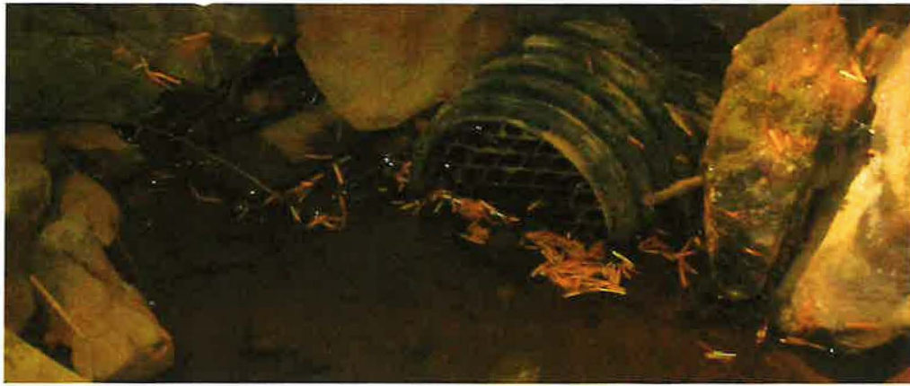
Intake with Fish Screen
