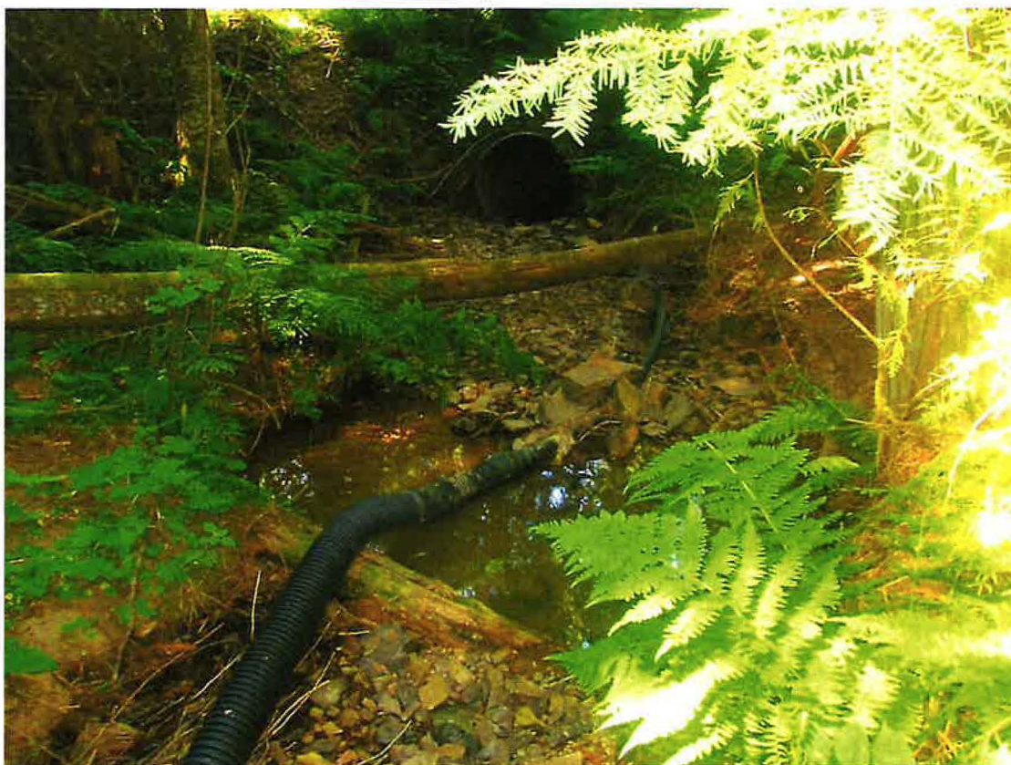
100 ft of corrugated pipe to 900 ft of 2-inch pipe to Pond
