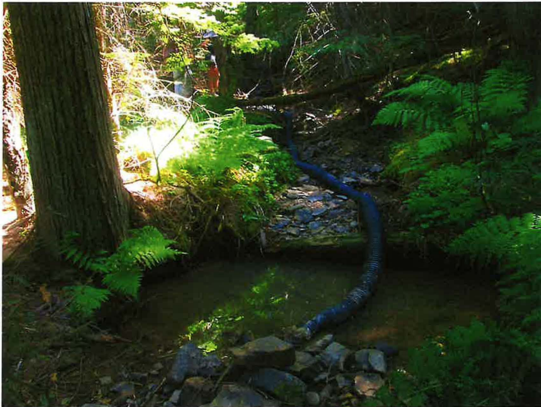
100 ft of corrugated pipe to 900 ft of 2-inch pipe to Pond
