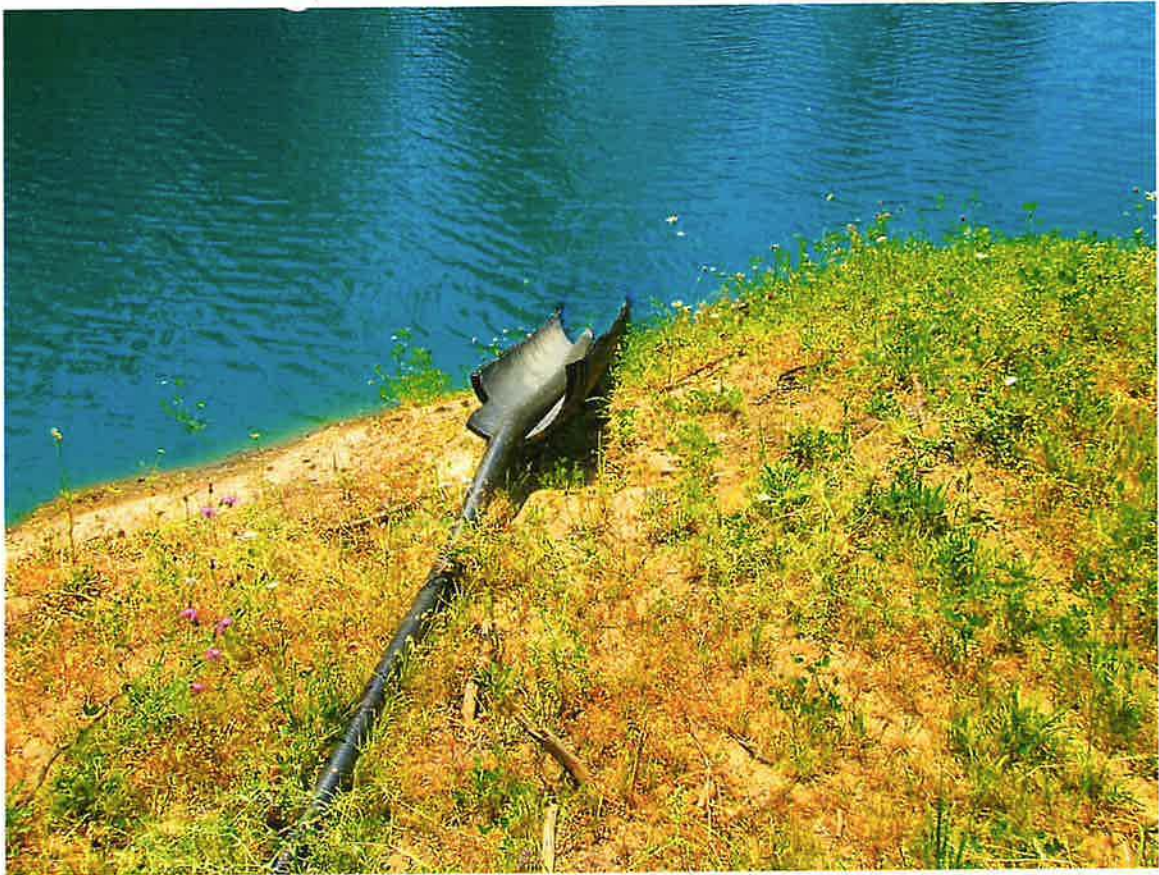
Outflow from Storage Pond to Pump House with Booster Pump to Irrigation System
