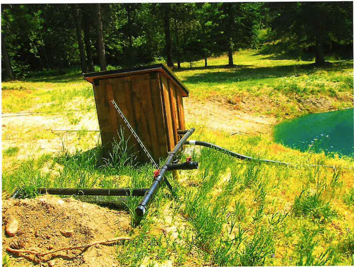
Outflow from Storage Pond to Pump House with Booster Pump to Irrigation System
