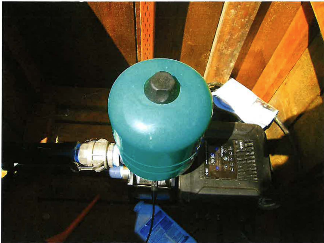
3 HP RPS Booster Pump & Sprinkler Manifold
