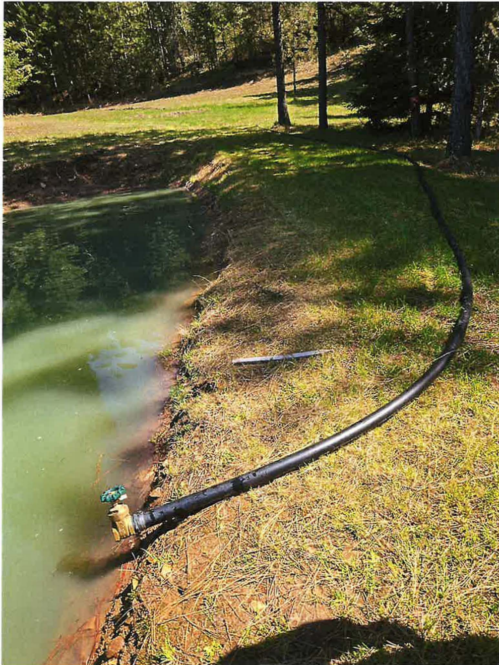
2 Inch Gravity Fed Line Diversion to Irrigation
