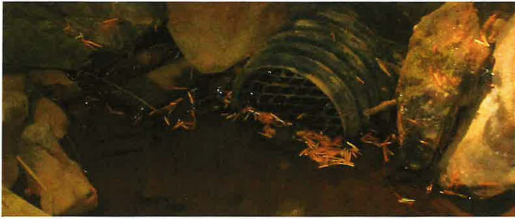
Intake with Fish Screen
