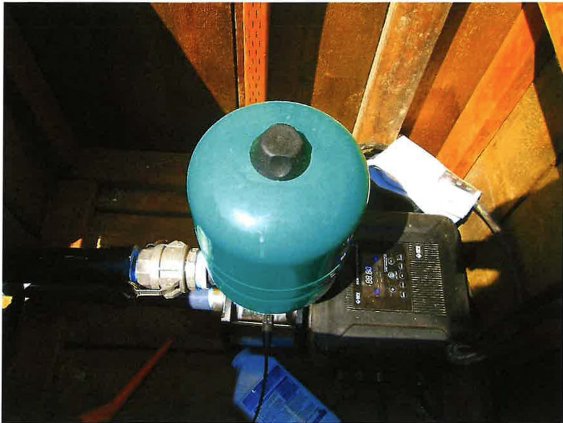
3 HP RPS Booster Pump & Sprinkler Manifold pulling from the Pond
