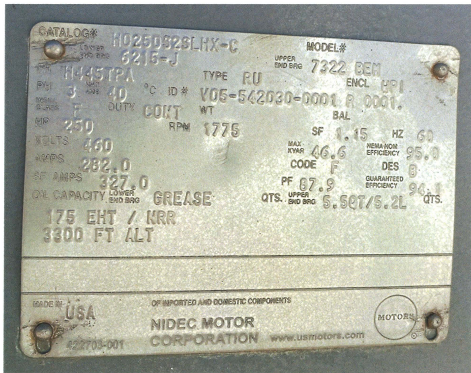
Figure 6 Motor specification tag for well D0057945.
