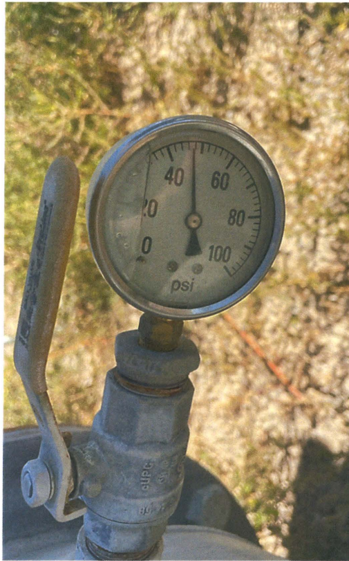
Figure 13 Pressure gage reading 48 psi for pump associated with well D0072831.
