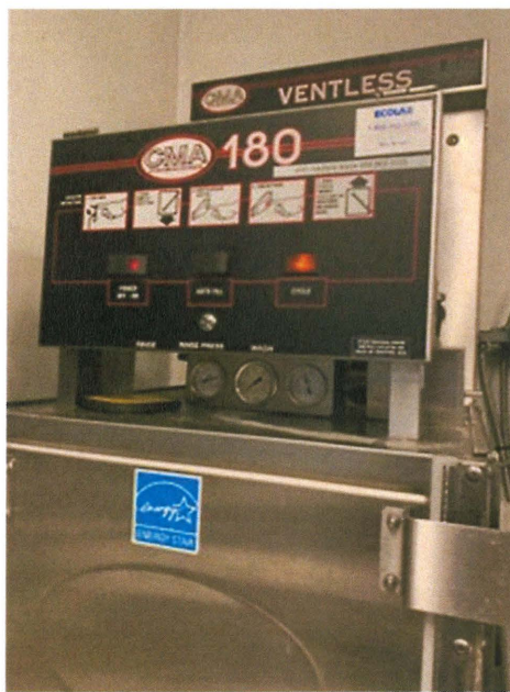
Figure 12 CMA 180 Ventless dishwasher by Ecolab used in kitchen.
