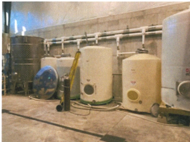
Figure 19 Four of thirty-five small fermentation tanks located in wine production facility.
