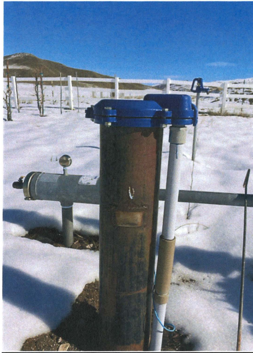
Figure 6 Well head for well D0082607.
