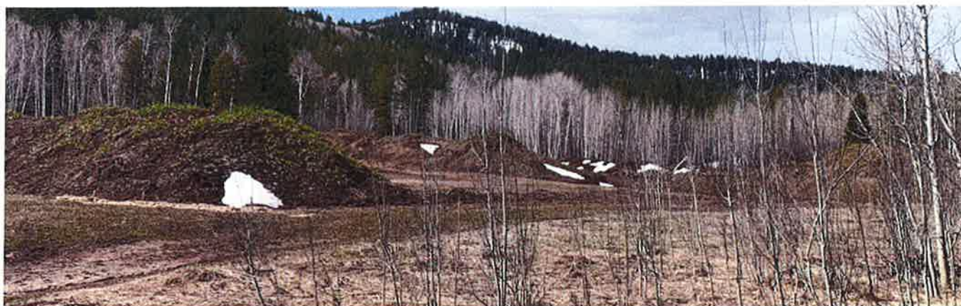
Figure 10. Photographic example of loose soil stockpiles in the background that lack silt fence or other devices to prevent additional mobilization of fines from the subject property, April 23, 2025.
