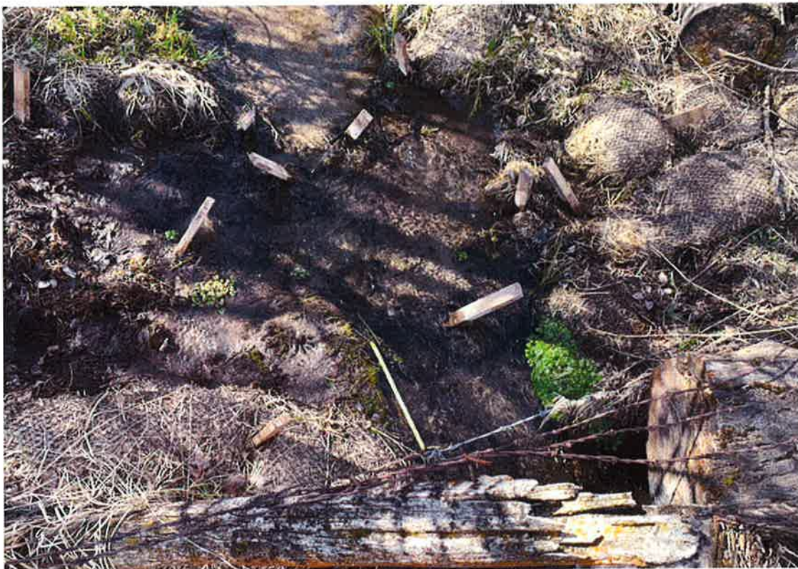
Figure 5. Photographic example of dilapidated straw wattles and the wooden stakes that used to hold them in place, at a location where surface waters exit the subject property within an altered spring creek stream channel, April 23, 2025.
