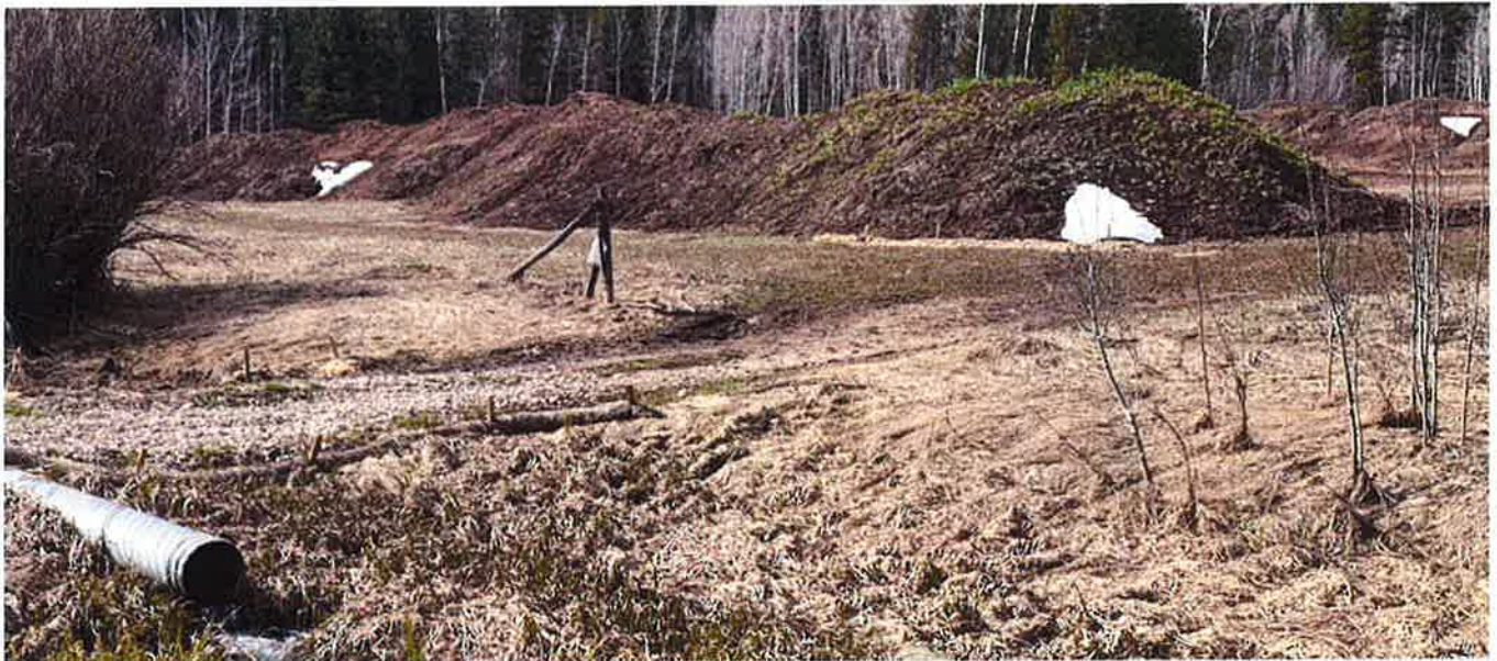
Figure 9. Photographic example of a loose soil stockpile that lacks silt fence or other devices to prevent additional mobilization of fines from the subject property, April 23, 2025. Note the photograph does depict about 20 ft of straw wattles installed at the base of the soil stockpile, but that wattle does not encircle the stockpile nor does it extend along the entire down-gradient extents of the stockpile.
