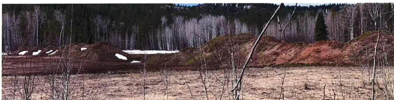
Figure 11. Photographic example of loose soil stockpiles and extensive area of vegetation removal and site disturbance that lack silt fence or other devices to prevent additional mobilization of fines from the subject property, April 23, 2025.
