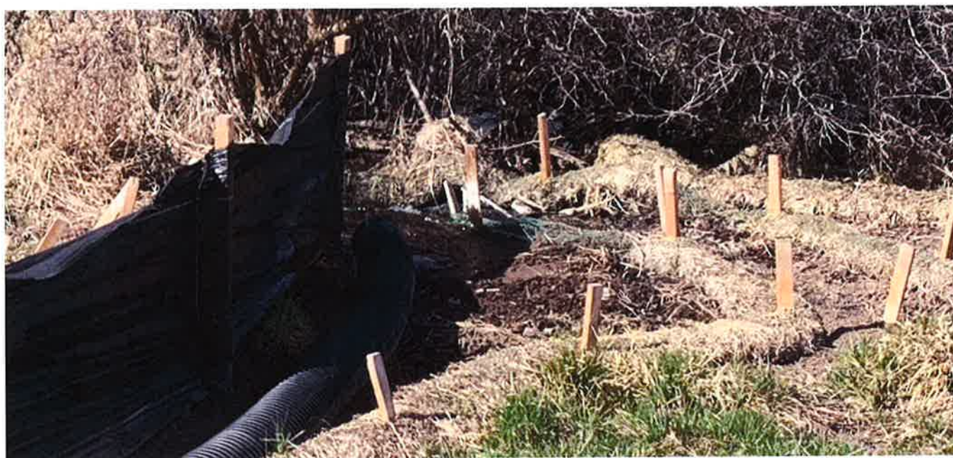
Figure 7. Photographic example of dilapidated straw wattles at a location where surface waters exit the subject property within an altered spring creek stream channel, April 23, 2025.
