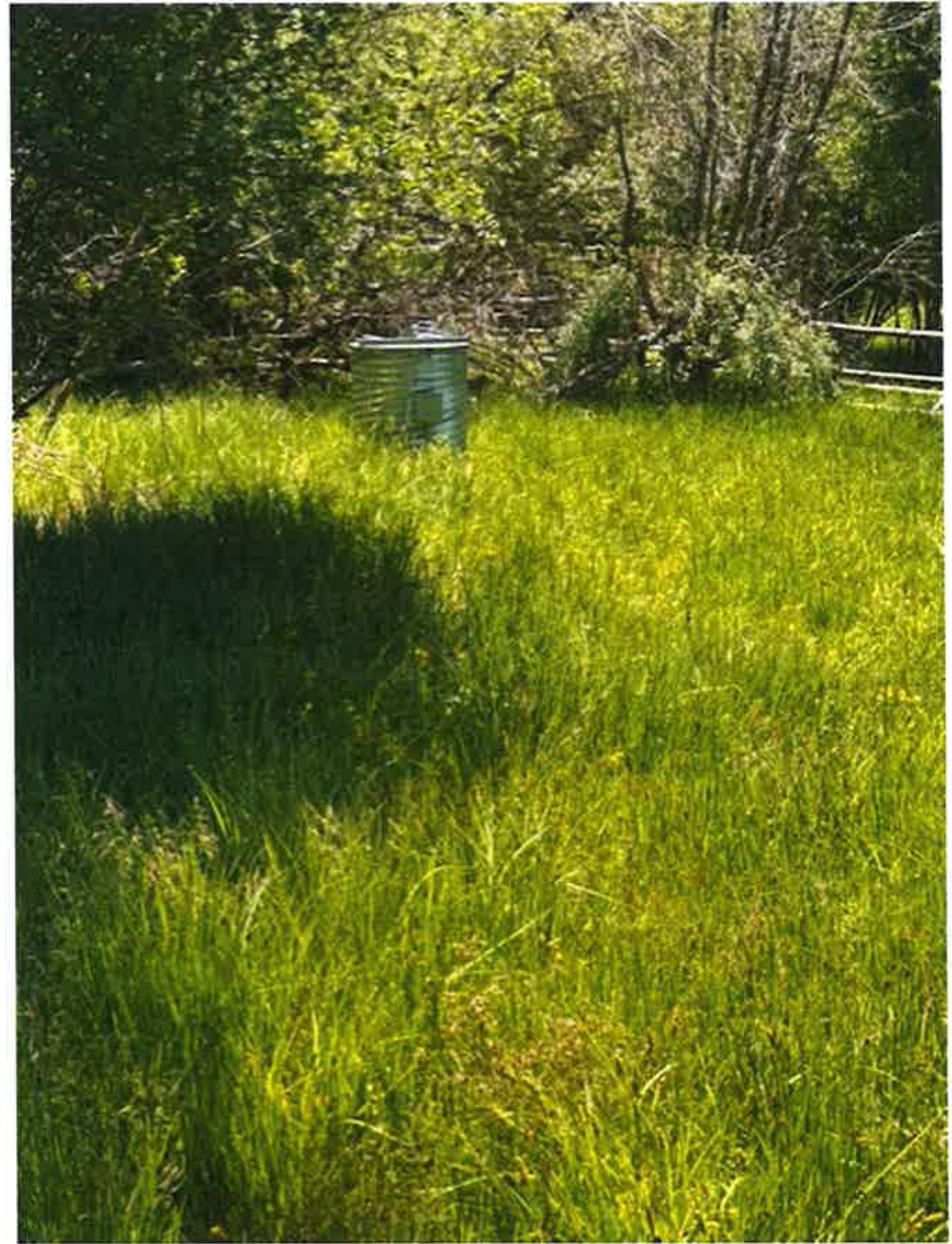
Spring box in corner of property. Pump in box.
