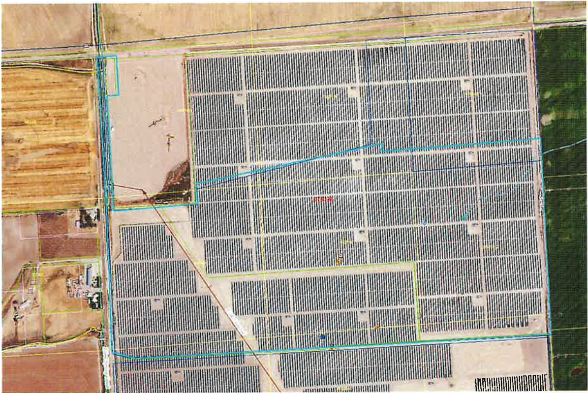
Figure 3- GIS 2017- Aerial Imagery of the parcels appurtenant to right 29-14015
