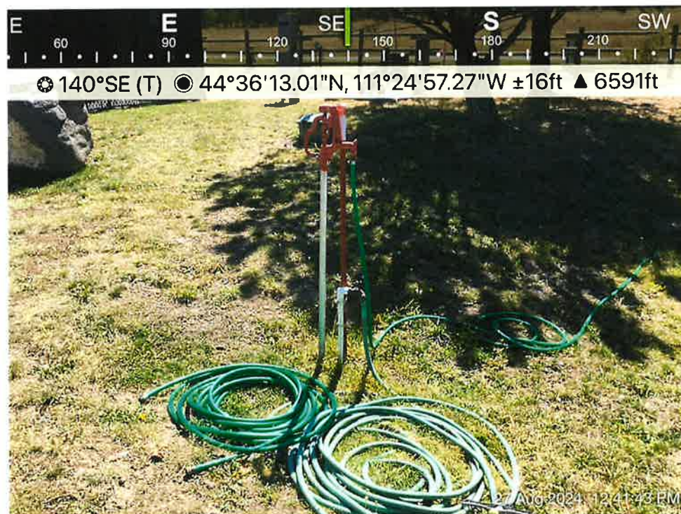
This is where they can tie in the 2 wells together
