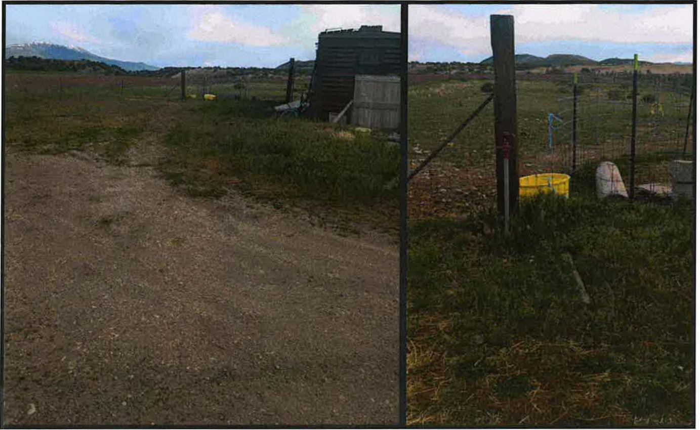
Figure 3. Stock water Pipeline Tee and Trough Hydrant, May 16, 2025.
