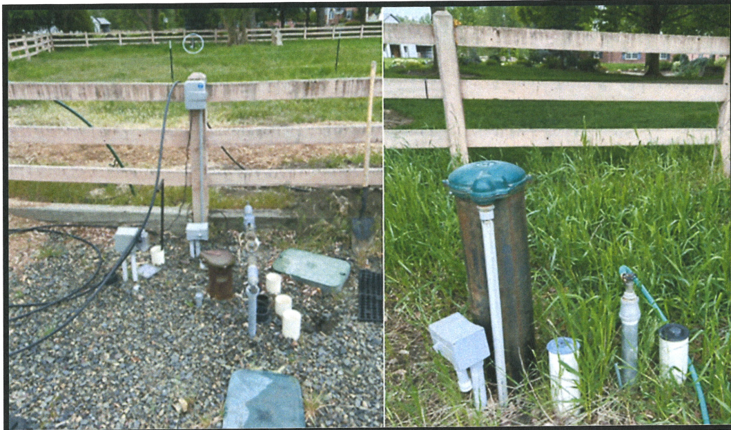
Photos 4 & 5- Standing north of the old well head (in left image) facing south with the new well head (in right image) in the background circled in blue.
