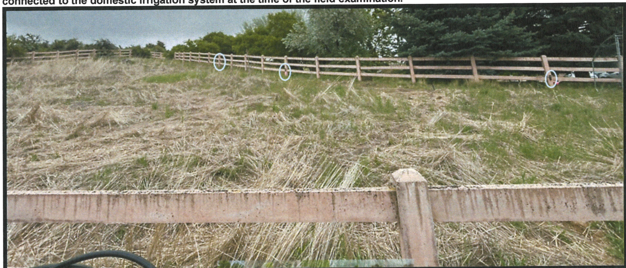
Photo 32- Triangular enclosure facing northeast. Some of the new Rain Bird 5000 sprinkler heads (circled in blue) are attached to the fence posts around the perimeter.
