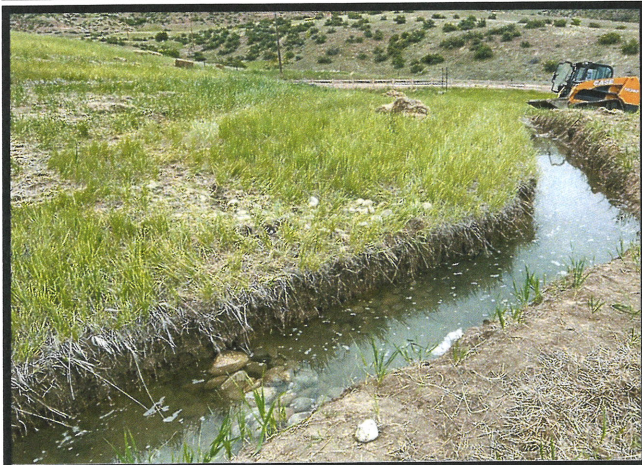
Photo 43, 44, & 45- Ditches intersecting the hillslope at 6' elevation intervals, approximately 25' downslope of each other.
