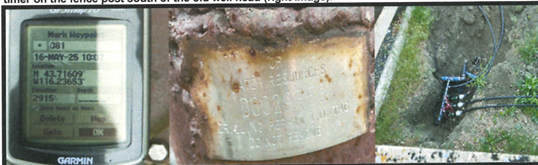
Photos 8, 9, & 10- GPS Coordinates (left image), well ID tag (center image) at the old well head, and control valves for garden driplines (right image) located on the west side of the fence surrounding the old well head.
