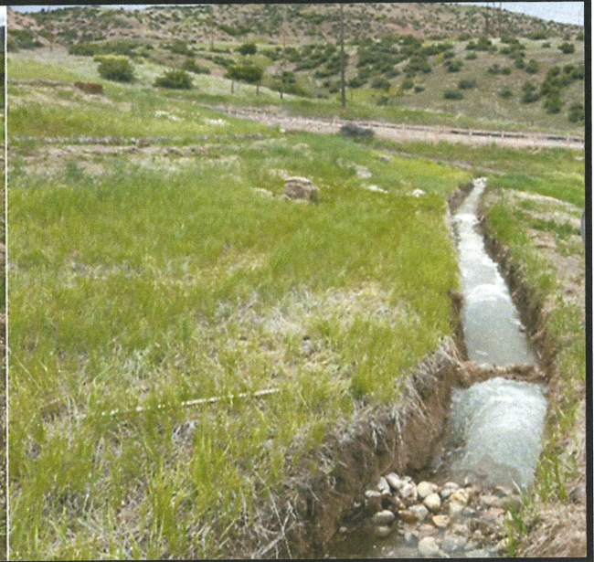
Photo 43, 44, & 45- Ditches intersecting the hillslope at 6' elevation intervals, approximately 25' downslope of each other.
