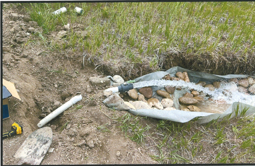
Photo 42- One of the 2" turnouts opened filling an irrigation ditch near the top of the hillside.
