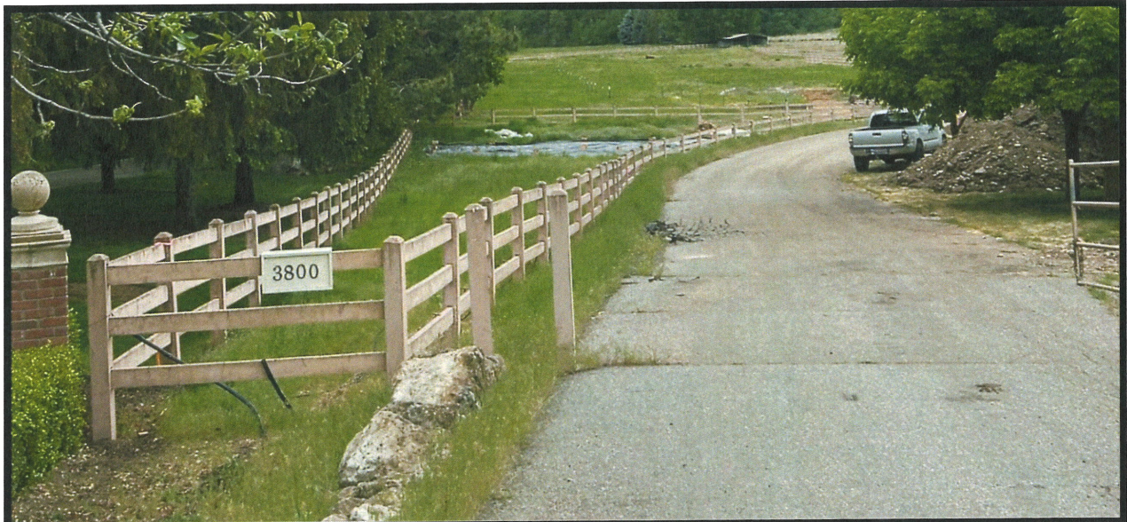
Photo 34- At the east end of the driveway facing west. The flower garden with driplines is installed in the fenced area on the left of the frame.
