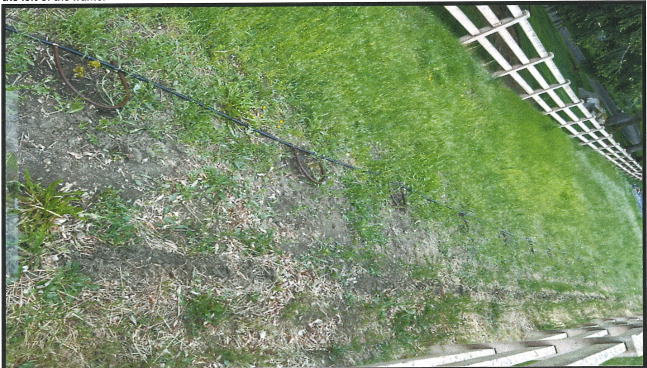
Photo 35- Driplines installed throughout the flower garden areas south of the driveway.
