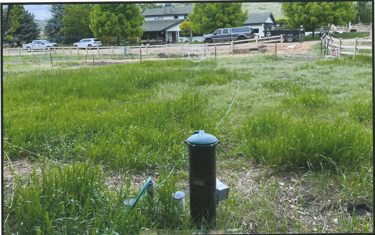
Photo 1- At the southern fence line facing north. The well POD in the foreground is south of the old well (circled in blue) where the new 2" PVC mainline connects to the old 1 1/2" PVC main to the "pump house" to the east of the home.
