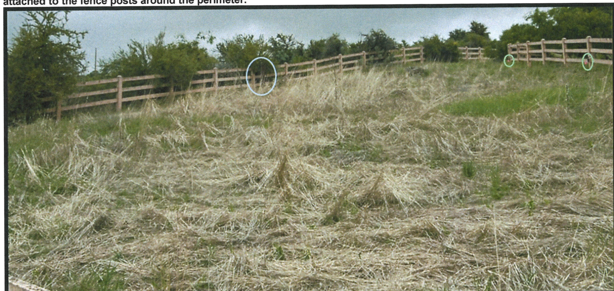
Photo 33- A vertical length of casing pipe midway along the western fence line (circled in blue) where a large rotary sprinkler was mounted to irrigate the triangular area. Several of the new Rain Bird 5000 sprinkler heads (circled in green) can be seen attached to the perimeter fence.
