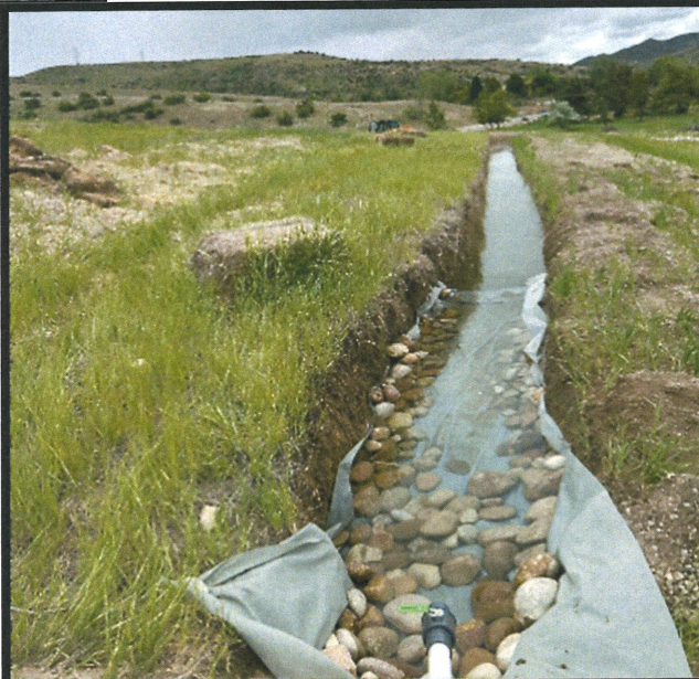
Photo 43, 44, & 45- Ditches intersecting the hillslope at 6' elevation intervals, approximately 25' downslope of each other.
