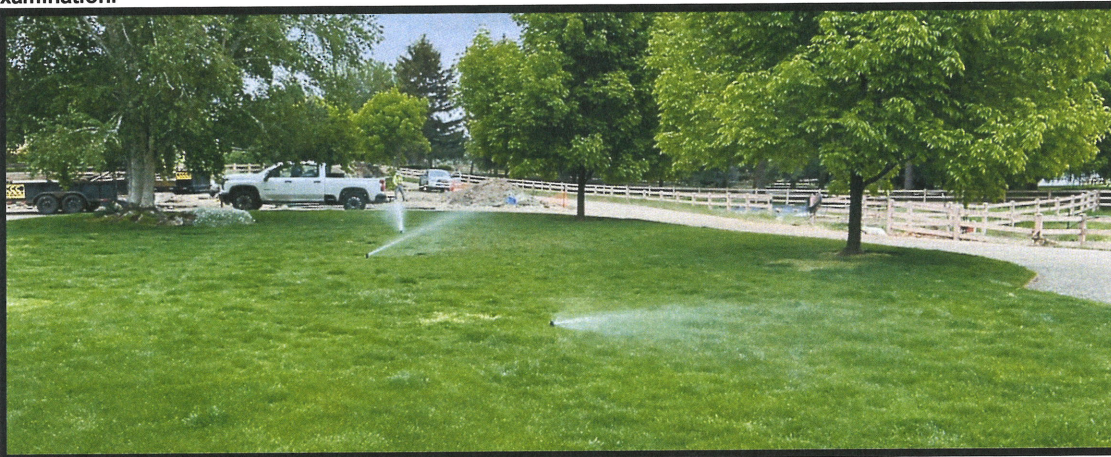
Photo 27- Domestic irrigation system zone in the southeast corner of the lawn with 7 sprinkler heads (Rain Bird 5000),
