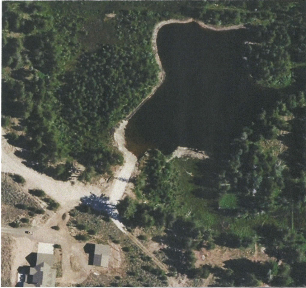
Figure 2 Aerial image of recreation storage pond provided by owner.
