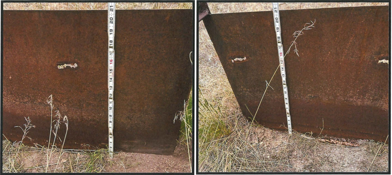
Photos 16 & 17- Standard tape measurements taken at the upstream (left image) and downstream (right) end of the weir. He MHW mark measured from about 8" to 9" in height.
