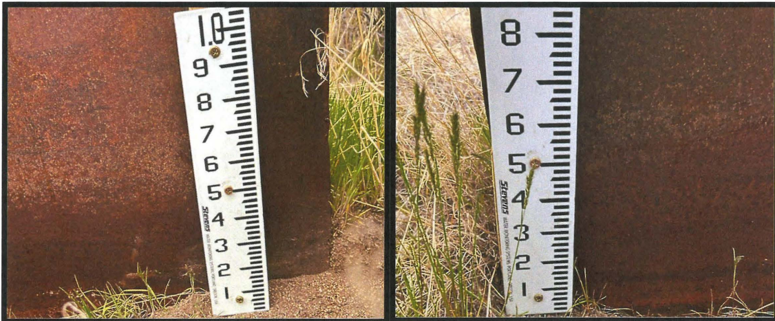
Photos 12 & 13- Staff gauge measurements taken at the east (upstream) end of the weir.
