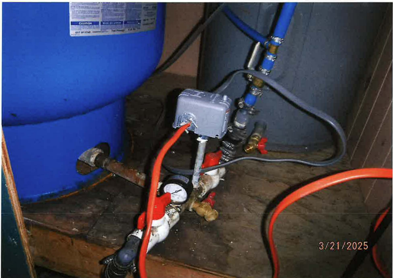
WATER CONVEYANCE SYSTEM – PUMP TO PRESSURE TANK TO BURIED POLY-PIPE MAIN SERVICE LINES TO THREE RESIDENCES & FROST-FREE HYDRANT(S)
