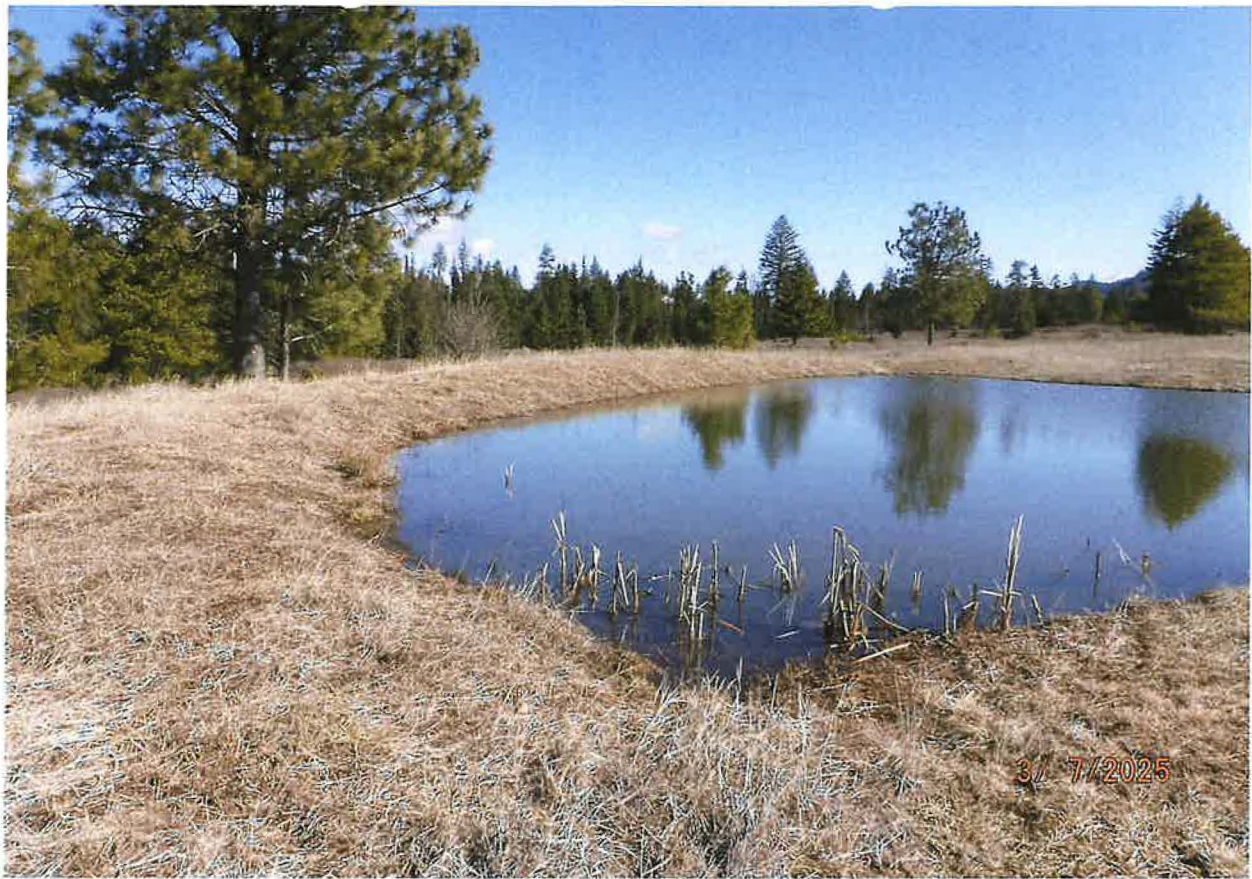
UPPER POND EARTHEN DIKE-DAM
