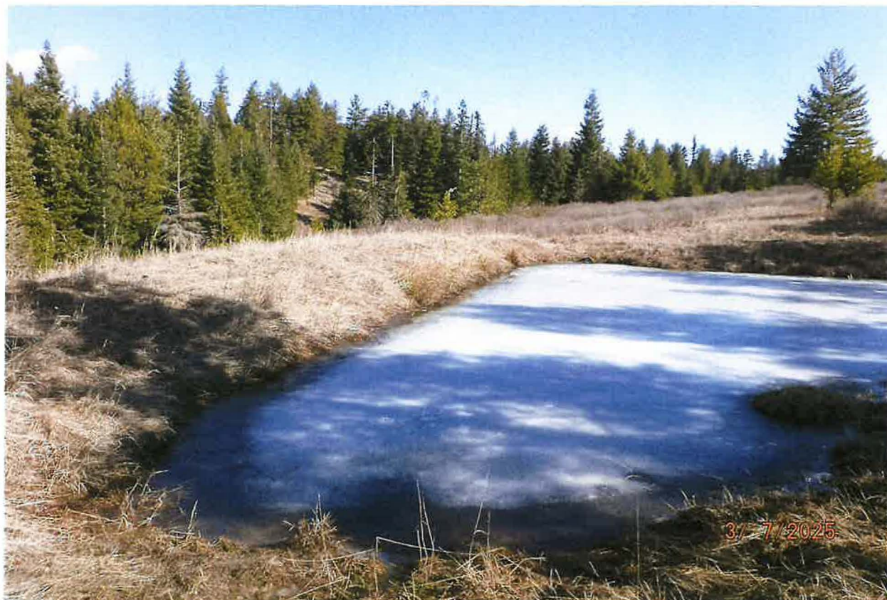
LOWER POND EARTHEN DAM-DIKE POD
