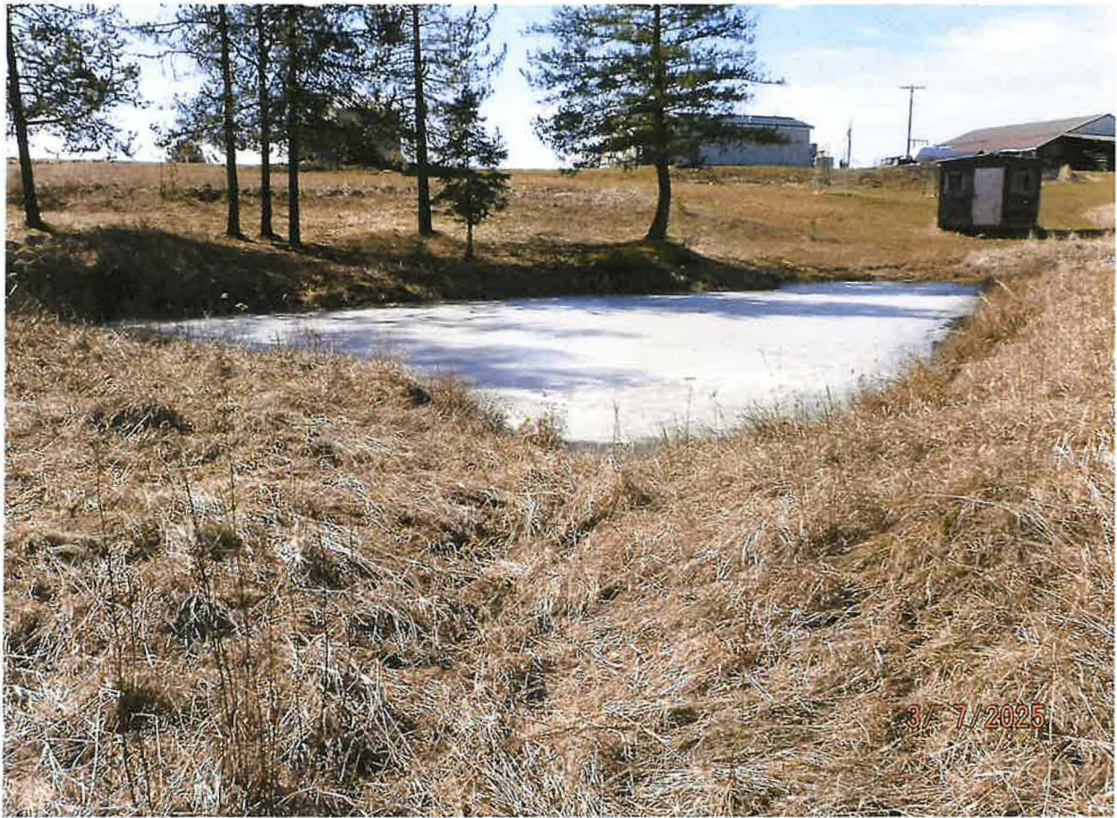
LOWER POND GRASSED OVERFLOW DISCHARGE CHANNEL
