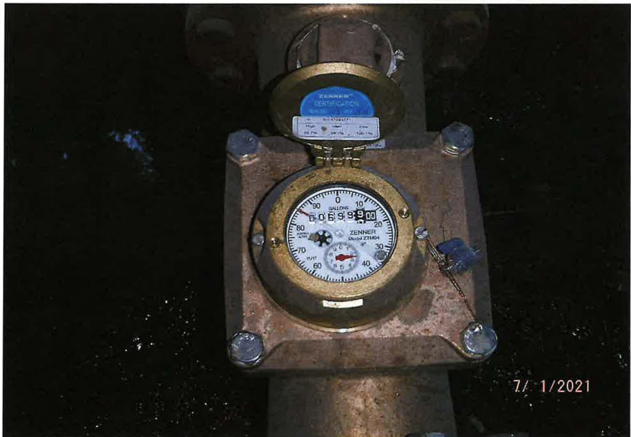
VELOCITY STYLE FLOW METER – ZENNER MODEL ZTM04 4-INCH FLANGED MOUNTING
