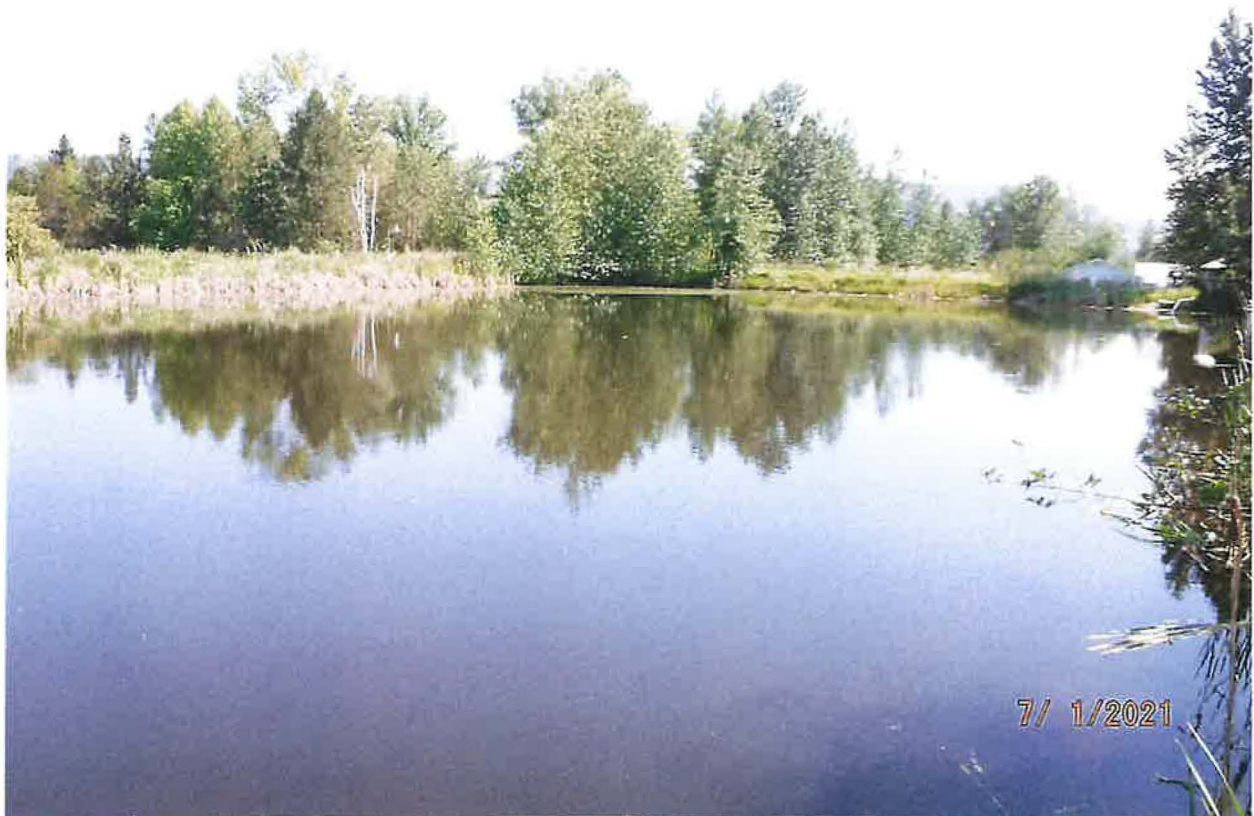
POU – POND #4 (MILL FIRE POND 1) INDUSTRIAL STORAGE & FIRE PROTECTION STORAGE – WATER IS PUMPED TO OTHER PONDS FOR INDUSTRIAL LOG WATERING FROM THIS POND
