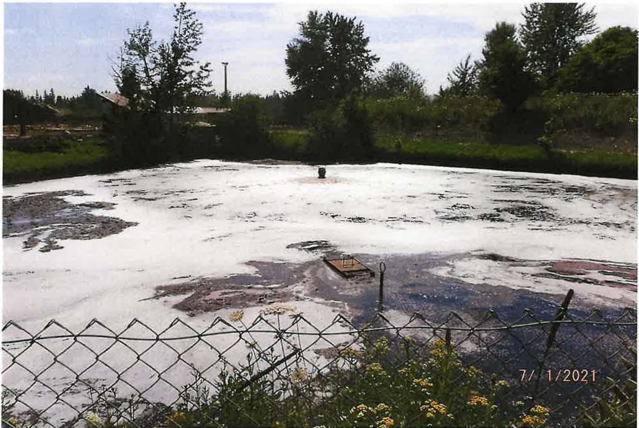
POU – POND #1 (SETTLING POND) INDUSTRIAL STORAGE & FIRE PROTECTION STORAGE – WATER IS RE-CIRCULATED FOR INDUSTRIAL LOG WATERING FROM THIS POND
