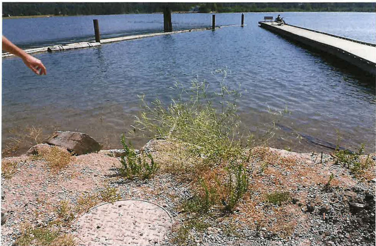
POD – PEND OREILLE RIVER DIVERSION; DUPLEX PUMP SYSTEM 2EA 10 HP PUMP TO SINGLE CONVEYANCE PIPELINE.
