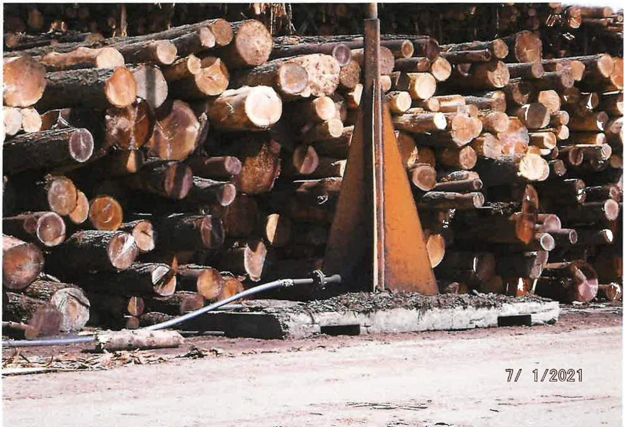
INDUSTRIAL FROM STORAGE POU – TRANSFER PUMPS TO BIG GUN WATER TOWERS FOR LOG WATERING
