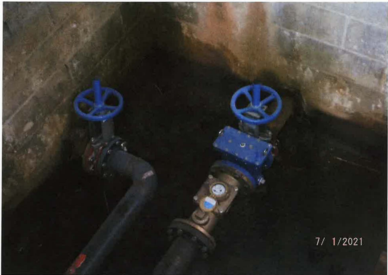
INFLOW LINE WITH FLOWMETER INSTALLED FROM PEND OREILLE RIVER
