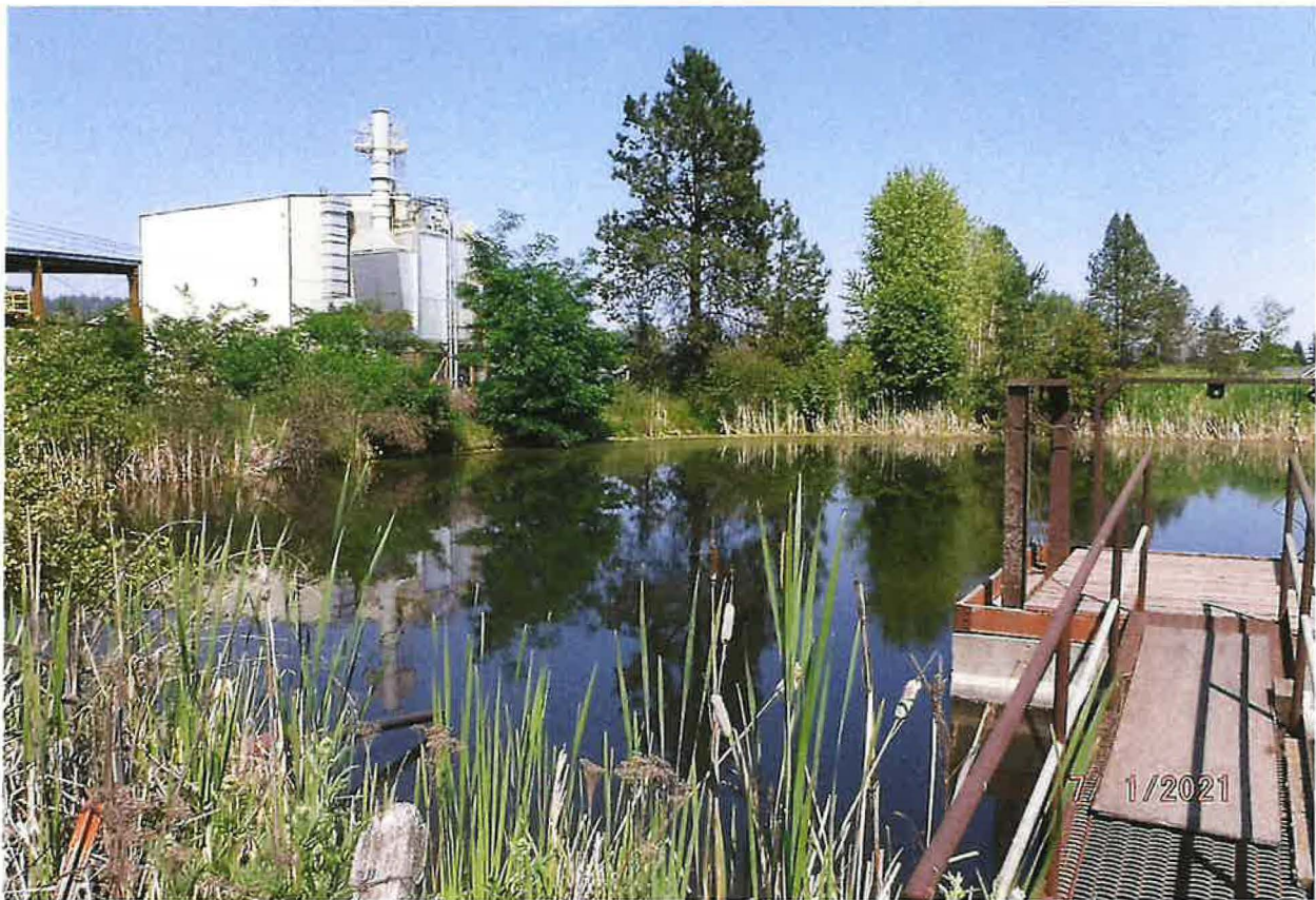
POU – POND #3 (MILL FIRE POND 1) INDUSTRIAL STORAGE & FIRE PROTECTION STORAGE – WATER IS PUMPED TO OTHER PONDS FOR INDUSTRIAL LOG WATERING FROM THIS POND
