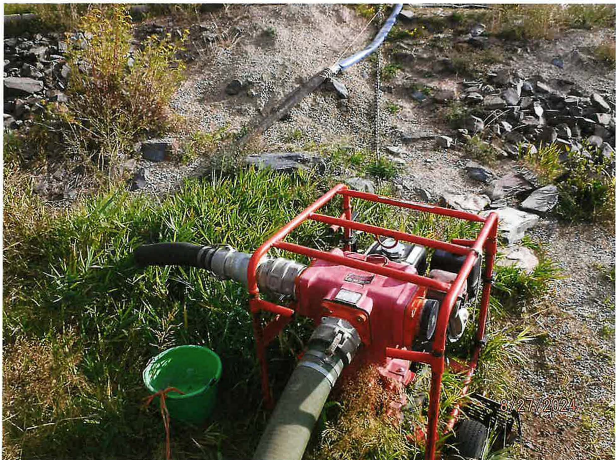
DIVERTING WORKS – GENERATOR MOUNTED WATER TRANSFER PUMP WITH 4-INCH DISCHARGE REDUCED TO 3-INCH FLEXIBLE ROLLED FIRE HOSE(S)
