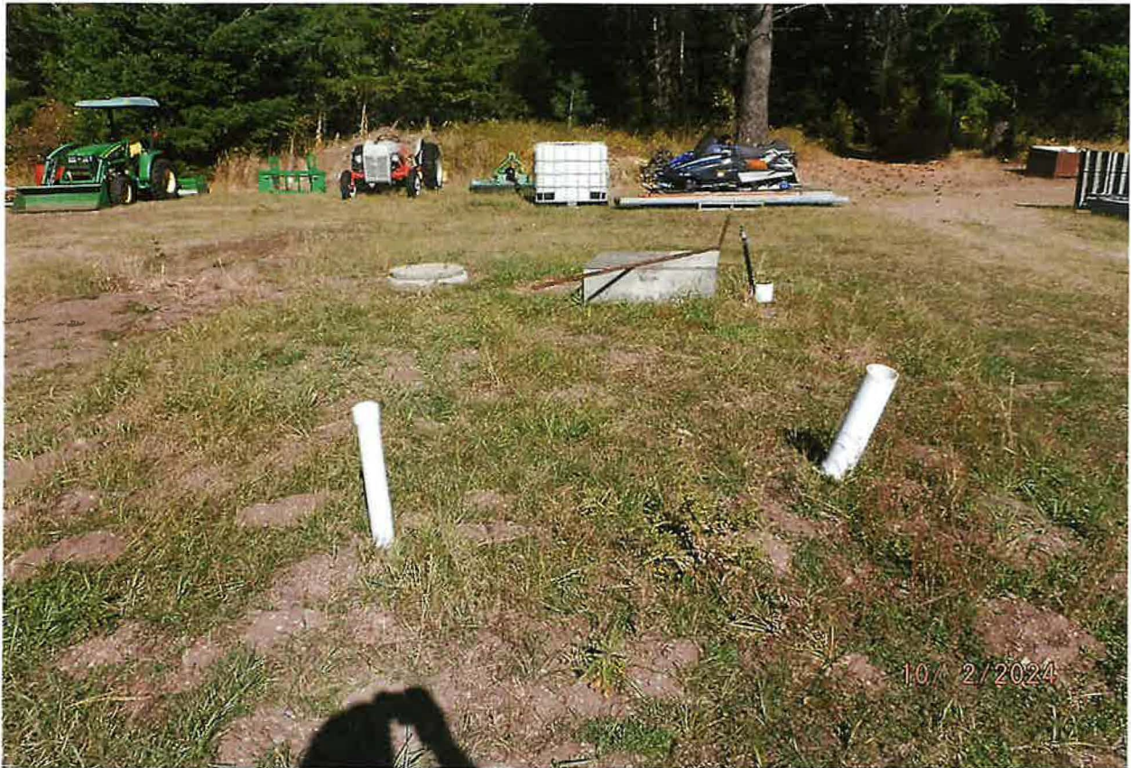
DOMESTIC POU – 2 RECREATION VEHICLE SERVICES, FULL WATER & SEWER CONNECTIONS WITH RESIDENTS USING FACILITIES THROUGHOUT THE YEAR
