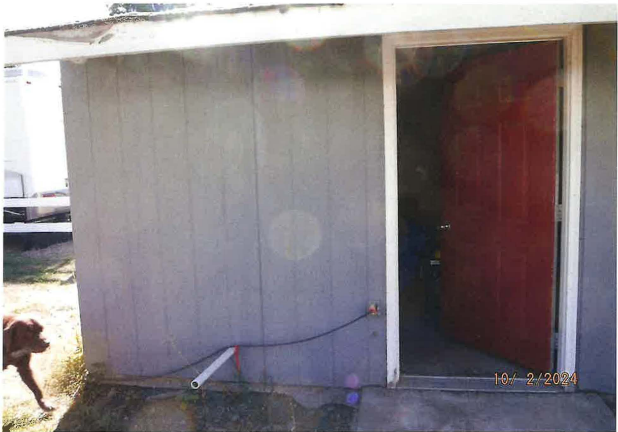
PUMP HOUSE CO-LOCATED WITH WELL
