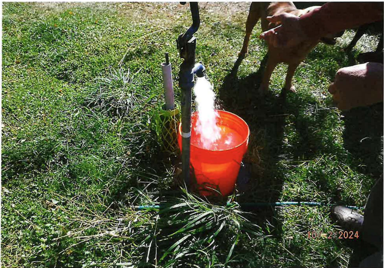
ONE OF EIGHT HOSE BIBS IN A LATERAL ROW RUNNING EAST/WEST ON THE PARCEL
