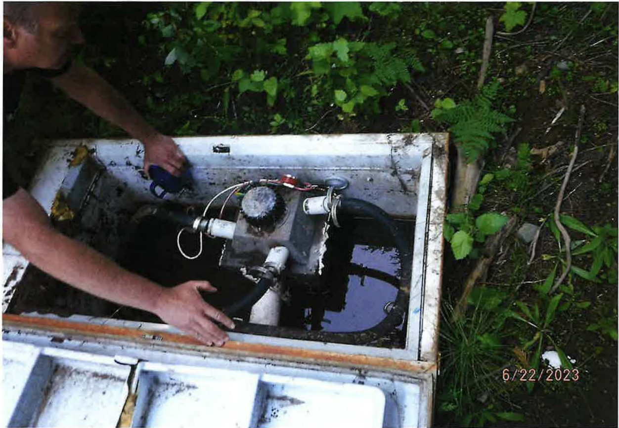
POU – POWER FROM STORAGE– POWER STATION INCORPORATES A REPURPOSED FREEZER HOUSING A MICRO-HYDRO SUPPRTORTING 3 NOZZLES (1/8", 3/16", & 1/4" NOZZLE SIZES)
