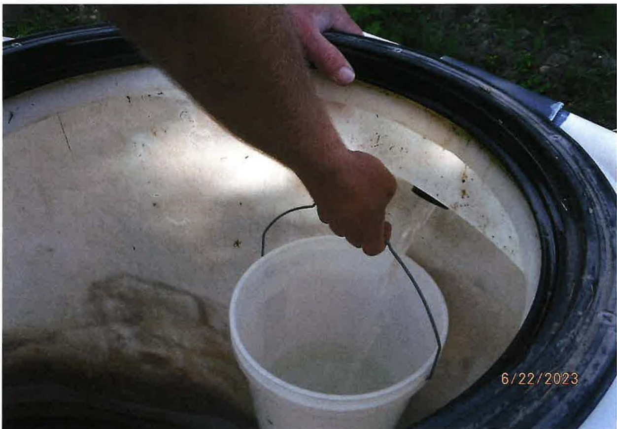
5 GAL BUCKET FLOW MEASUREMENT TAKEN AT INFLOW FROM SPRING CISTERN TO STORAGE TANK; 5 GAL BUCKET FILLED IN 39.14 SECONDS.
