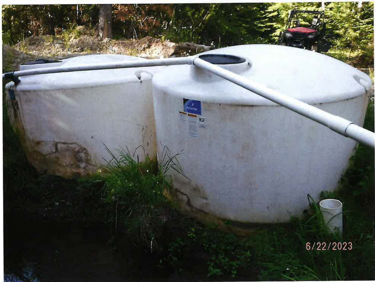
OVERFLOW PIPE FROM STORAGE TANKS CONVEYS EXCESS SPRING WATER DIRECTLY TO STORAGE POND
