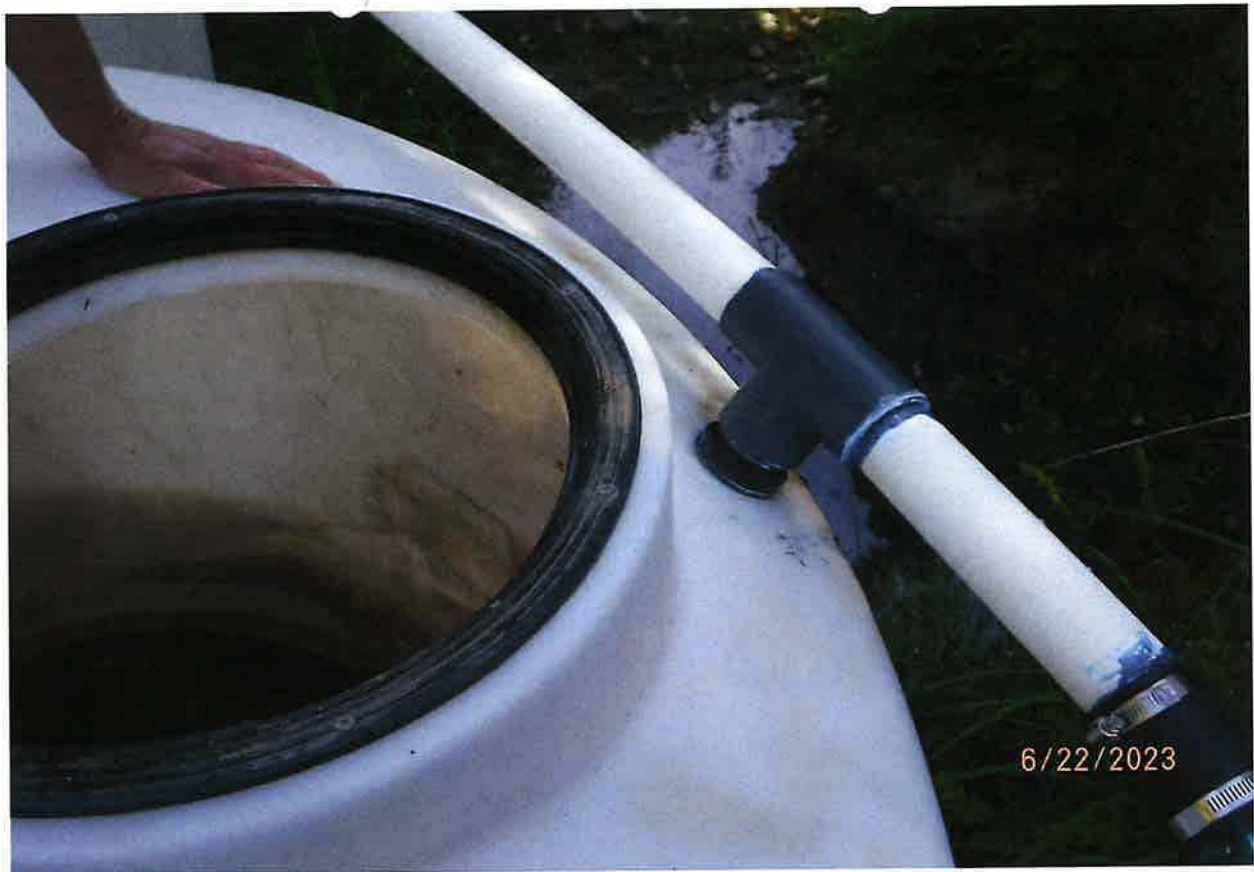
OVERFLOW PIPE FROM STORAGE TANKS CONVEYS EXCESS SPRING WATER DIRECTLY TO STORAGE POND
