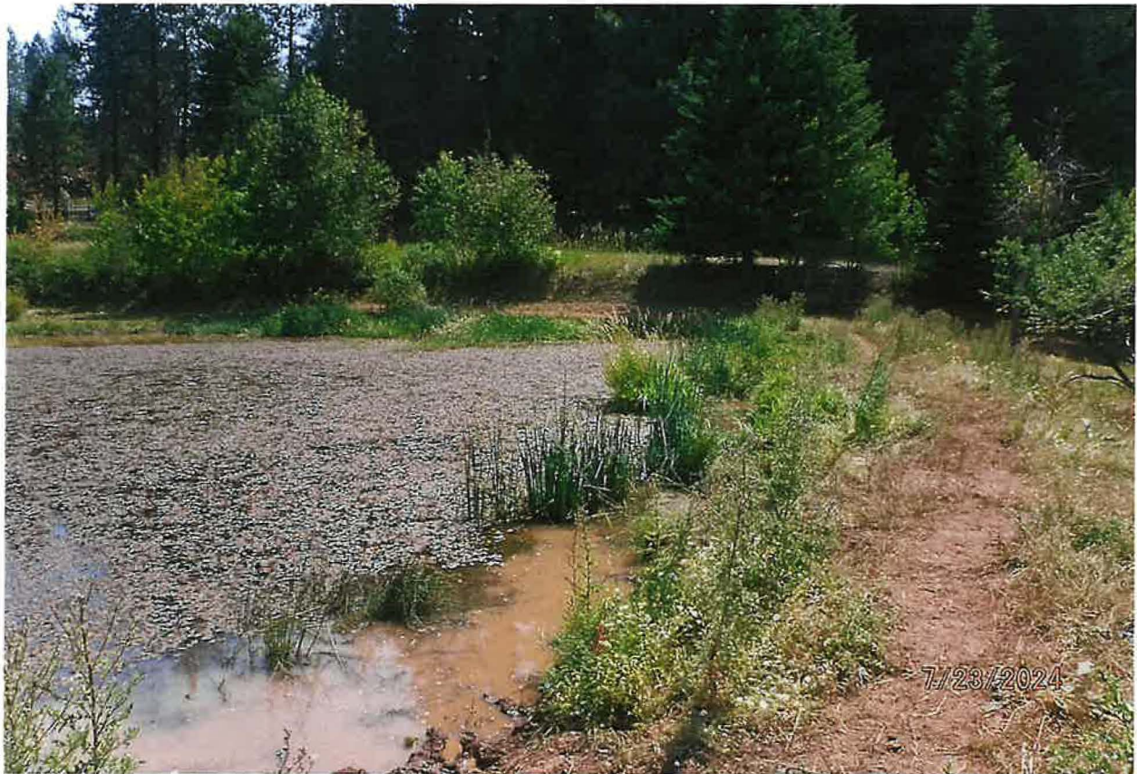
POD – EARTHEN DAM DIKE IMPOUNDS UNNAMED STREAM WATER
