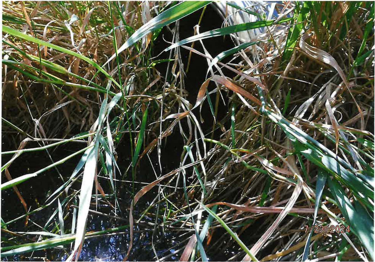
POD – EARTHEN DAM SERVES AS DRIVEWAY DIKED IMPOUNDING UNNAMED STREAM WATER. 24-INCH CULVERT ALLOWS OVERFLOW DISCHARGE WATER TO CONTINUE DOWNSTREAM
