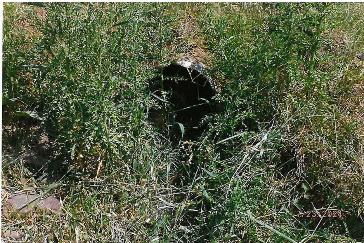
LOWER POND OVERFLOW DISCHARGE DOWN SLOPE VIEW – DRY AT TIME OF EXAM IN JULY
