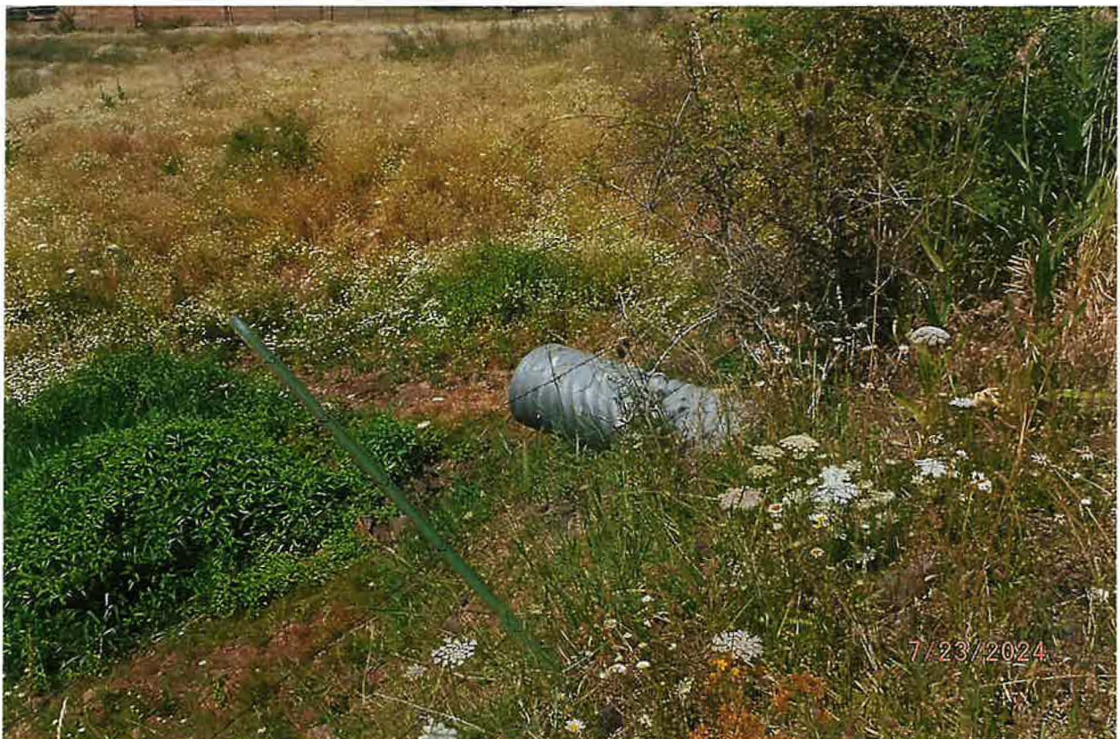
OVERFLOW DISCHARGE FROM UPPER POND – STREAM FLOW NORMALLY DRIES UP BY EARLY JULY EACH YEAR
