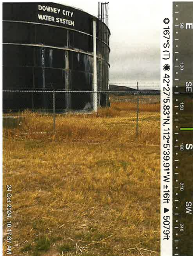
Water Tower spill pipe
