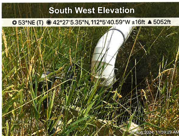
diversion into system
