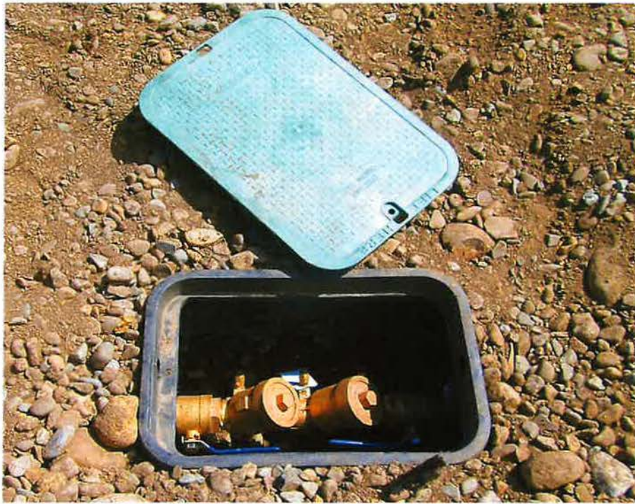
Sprinkler manifold & Well
