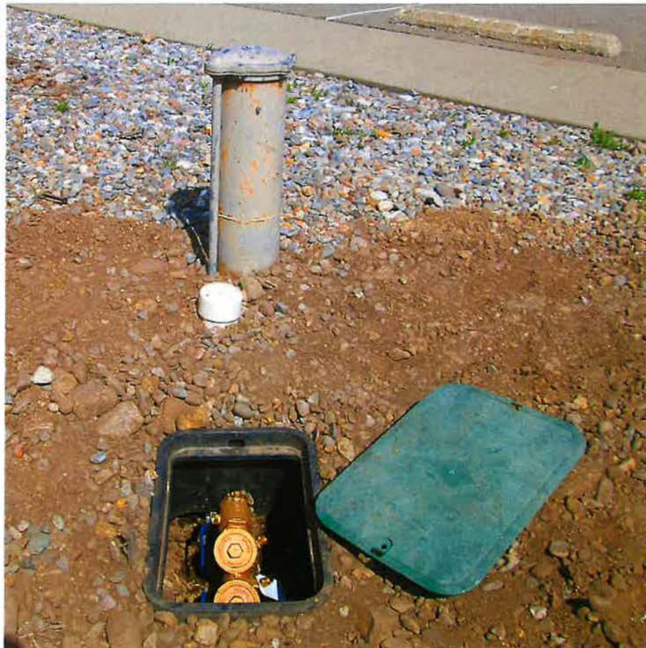
Sprinkler manifold & Well
