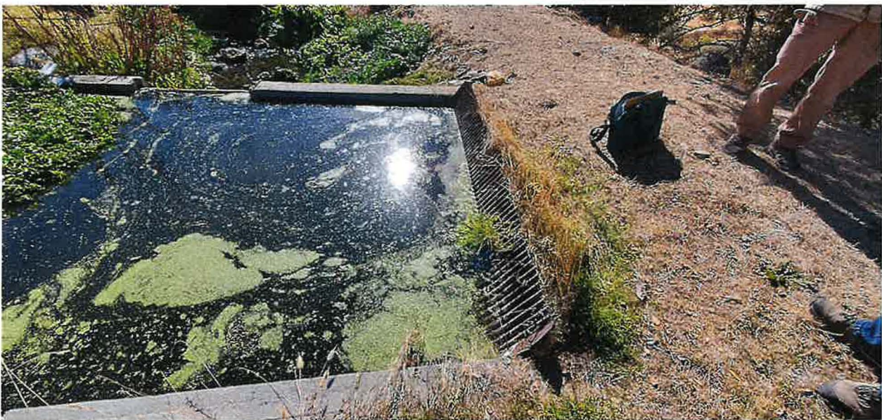
Figure 2: Top of penstock
